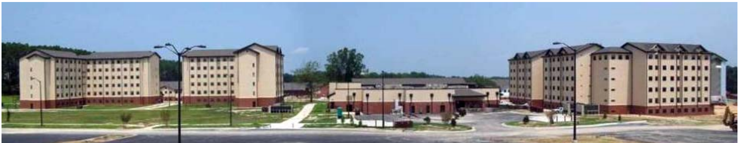
Phase one (pictured here) was completed August 2009 and includes two barracks, two headquarters, a dining facility and a COF. Top of page: barracks under construction. Photos provided by Steven G. Smith, project engineer.
