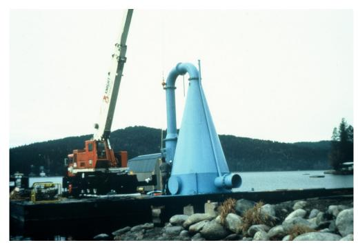
Figure 4-1 Speece Cone Being Installed in Newman Lake (from <u>www.eco2tech.com</u>)
