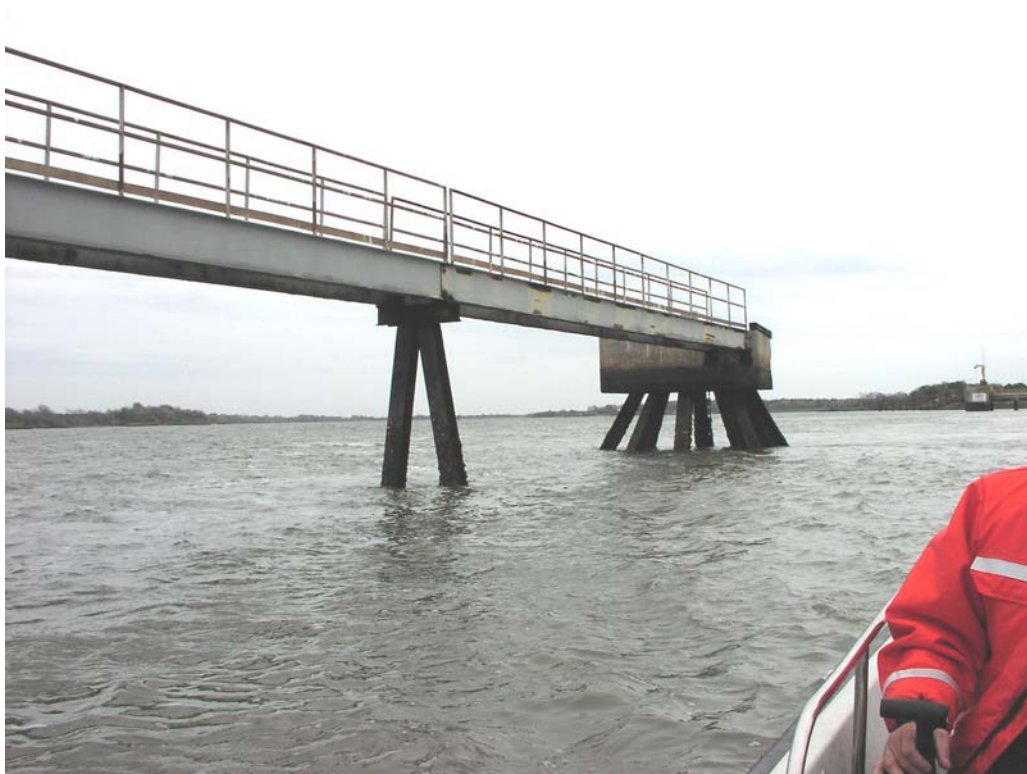
Kemira Inc. Dock and Pier. Stations 57+000 to 58+000, Foundation – Good Condition, Looking Downstream
