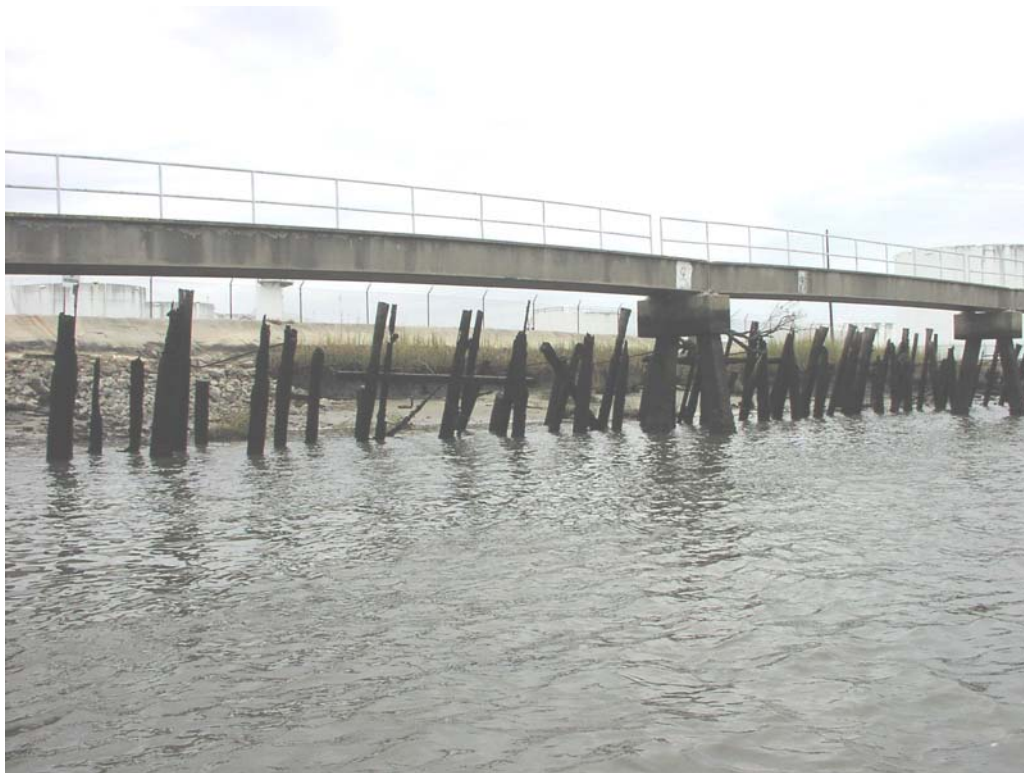
Unocal, Concrete Piles, Station 61+100, Good Condition
