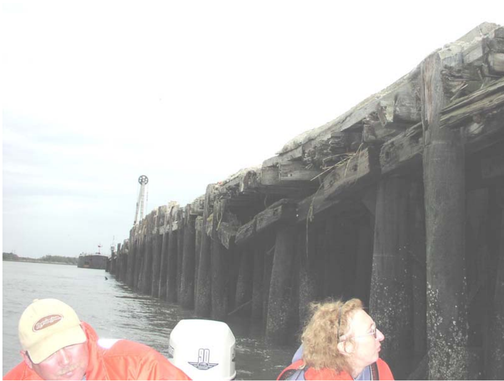
East Coast Terminal, Station 68+500, Wood Piling, Berth 4, Deteriorated/Broken Condition
