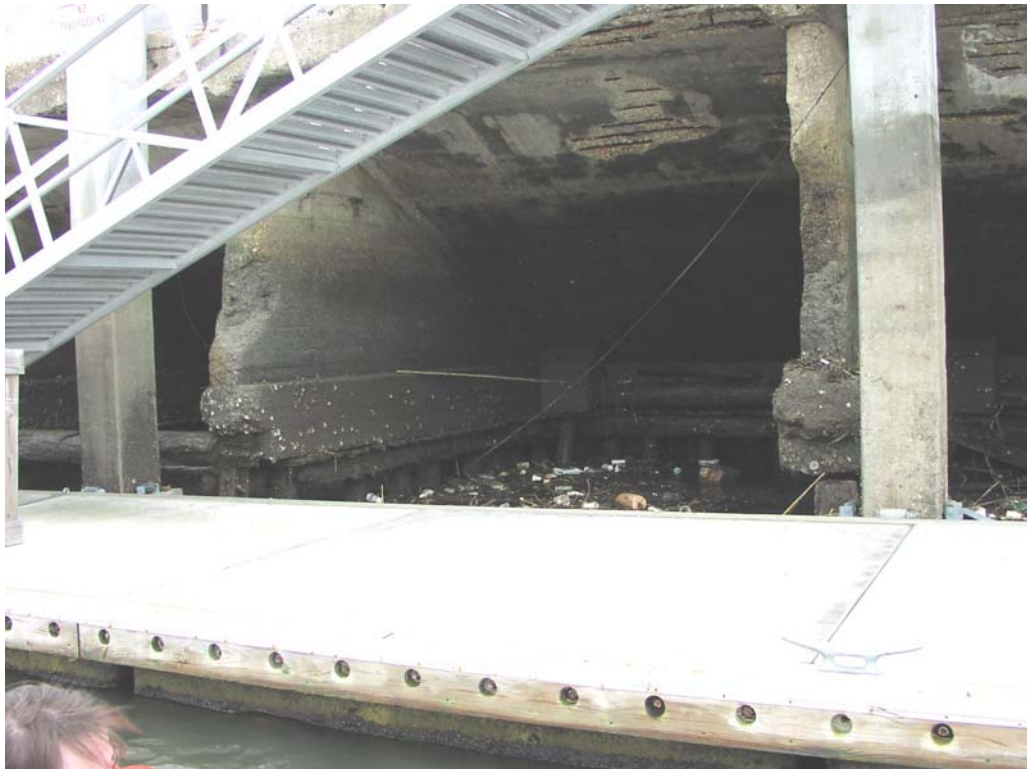
Parking Lot/Ferry Dock, Concrete Support on Wood Piles, Station 74+600, Poor Condition Note: Several to many wood piles not in contact with concrete support(s), Elevation ~1 MLW.
