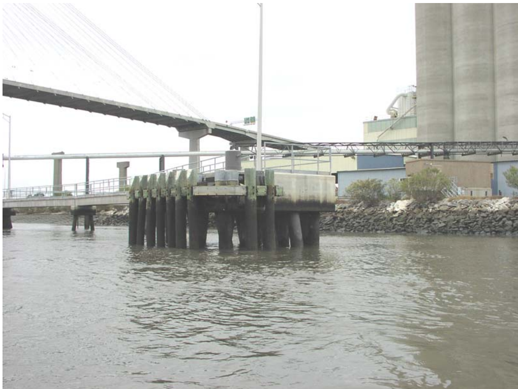
Blue Circle Cement, Approx. Station 78+550, Steel Shell Piles, Excellent Condition
