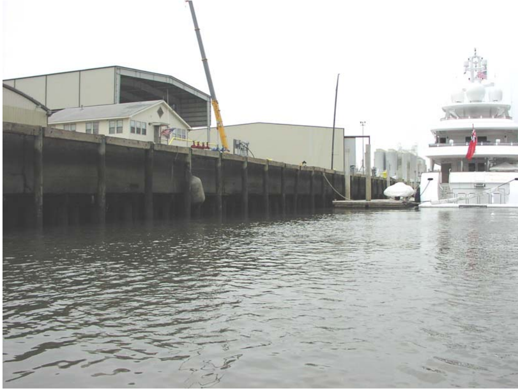
Intermarine, Station 83+900, Dock and Piling in Good Condition
