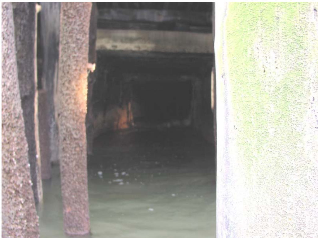
East Coast Terminal, Station 68+100, Wood Piling, Berth 4, Deteriorated/Broken Condition
