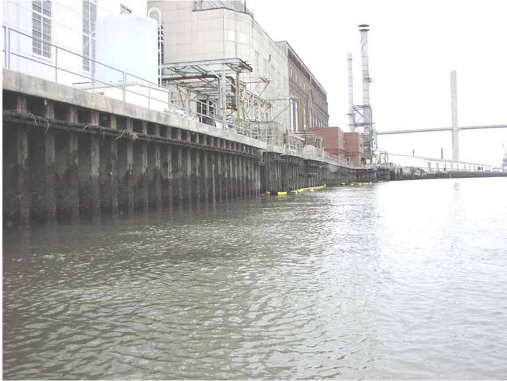
Savannah Electric Peaking Plant, Station 77+000, Good Condition
