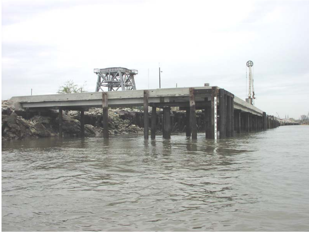
Standard Concrete Products, Steel Piles, Station 62+700, Good Condition
