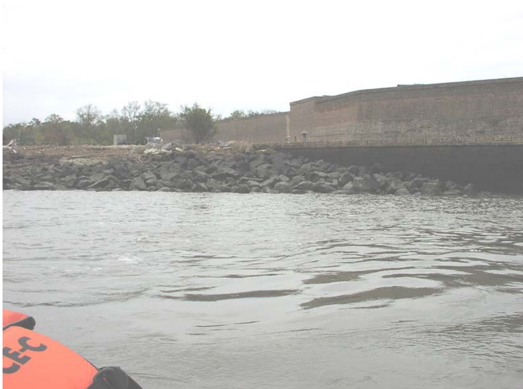
Old Fort Jackson, Downstream RipRap, Station 58+500
