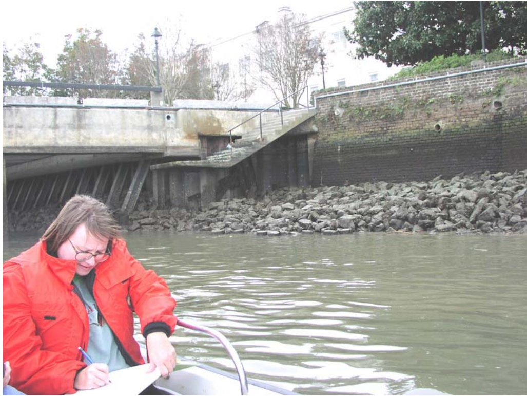
River Street, Station 74+800
