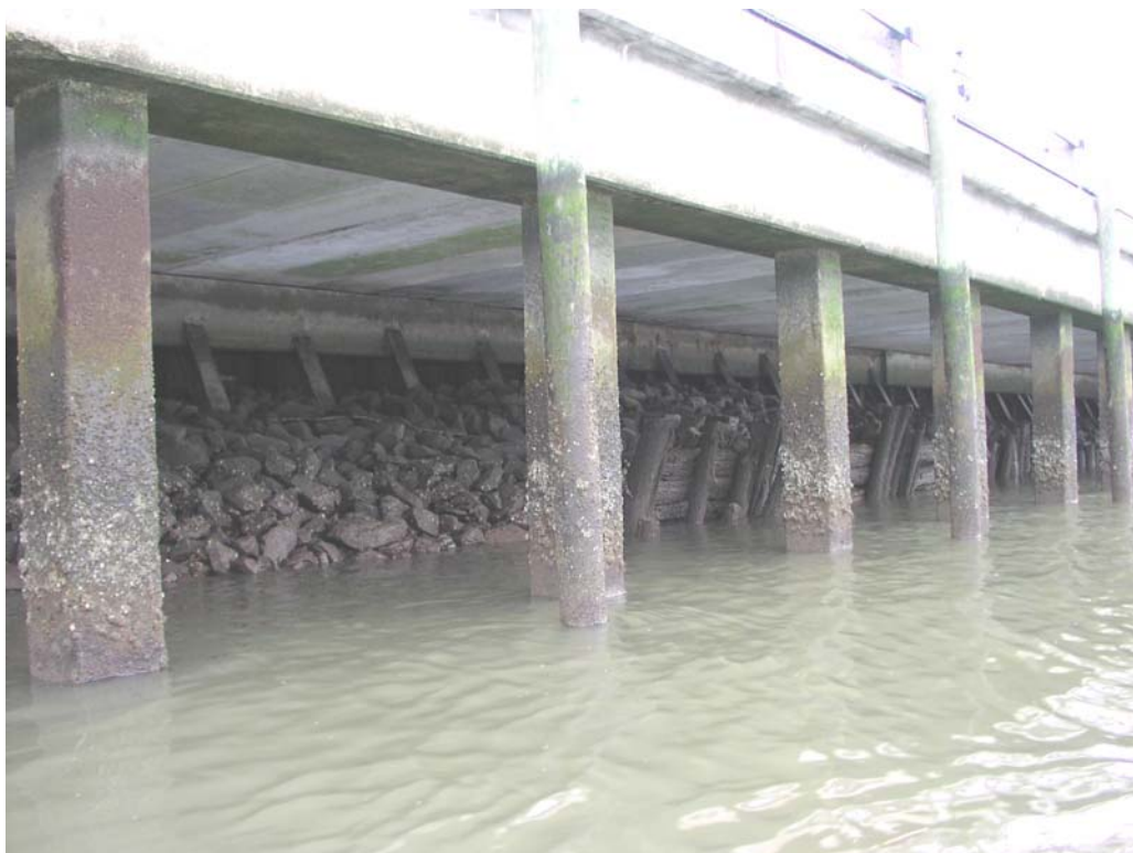
River Street, Approximate Station 75+200, Concrete and Steel Piling, Good Condition City Hall Area
