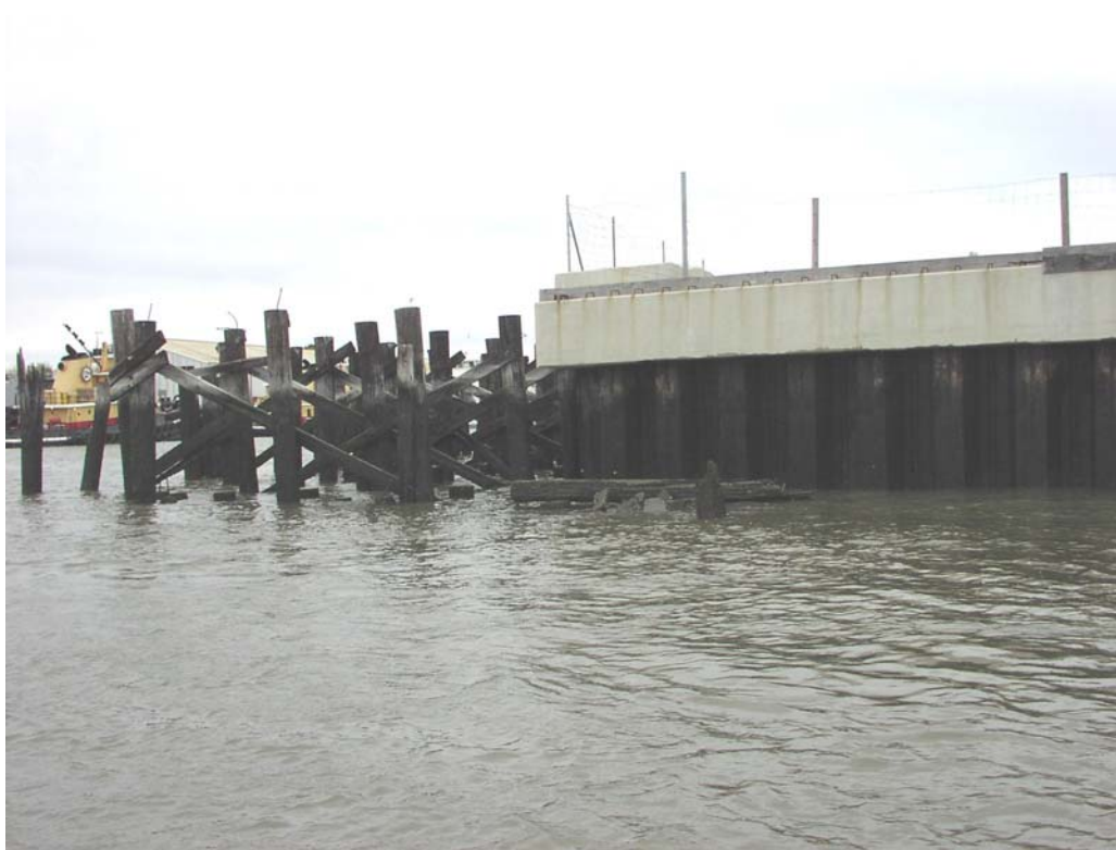
Convention Center, Steel Sheet Piles, Station 75+000, Good Condition
