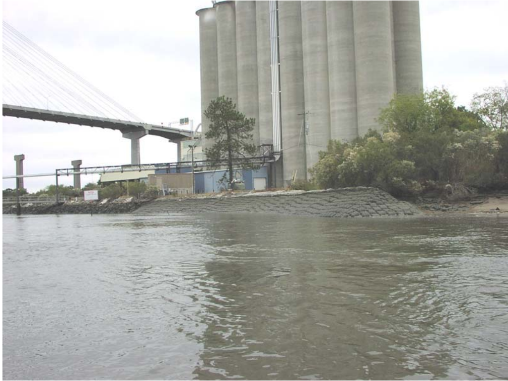
Blue Circle Cement, Approx. Station 78+300
