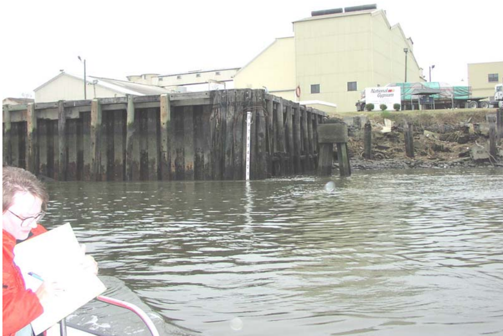
Georgia Kaolin Terminals, Station 90+700, Steel Sheet Piles, Good Condition
