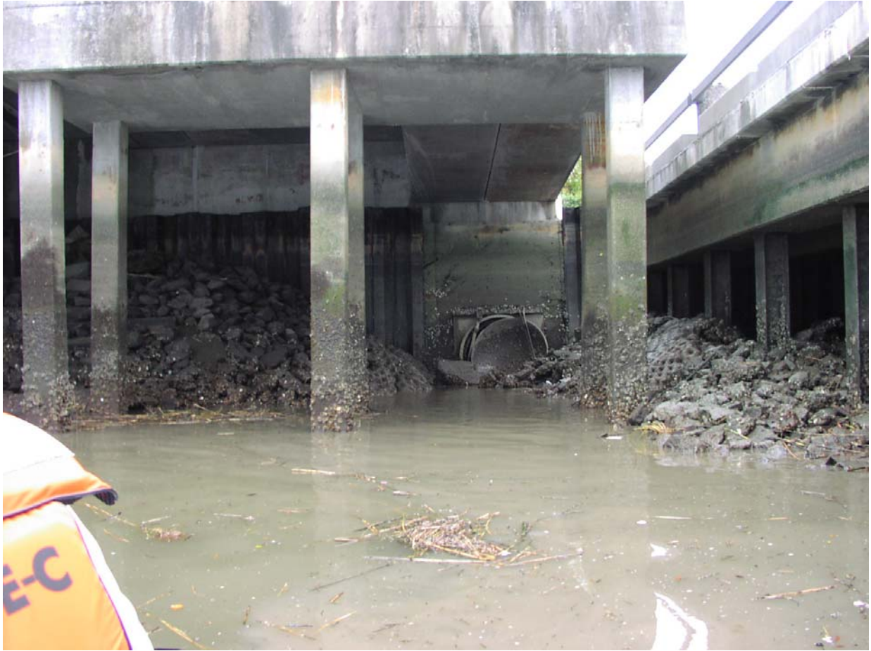
Marriott Hotel, Concrete Piles, Station 72+500, Good Condition Note blocked and broken flap gate at drainage pipe
