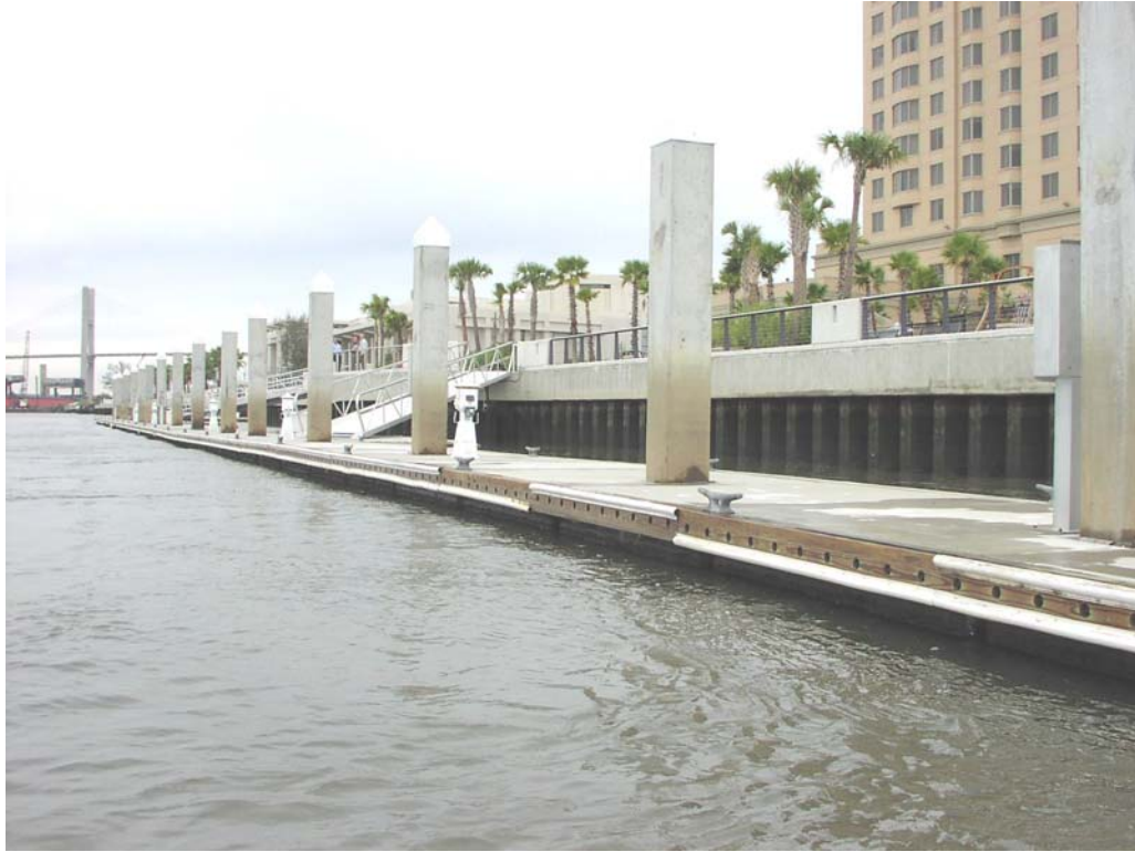
Weston Hotel, Steel Sheet Piles, Station 74+500, Good Condition
