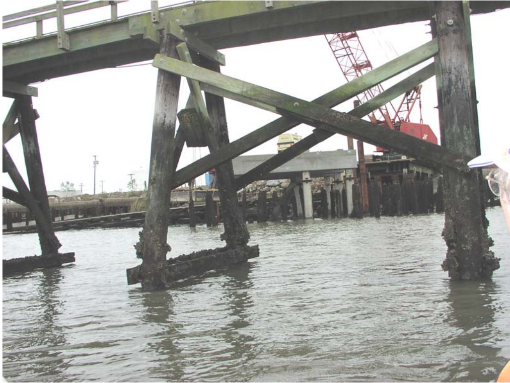
ST Services #2, Station 62+200, Wood Piles, Fair Condition
