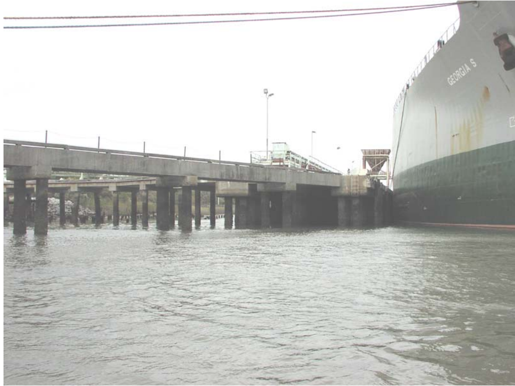
Georgia Pacific Gypsum, Station 63+250, Concrete Piles, Good Condition
