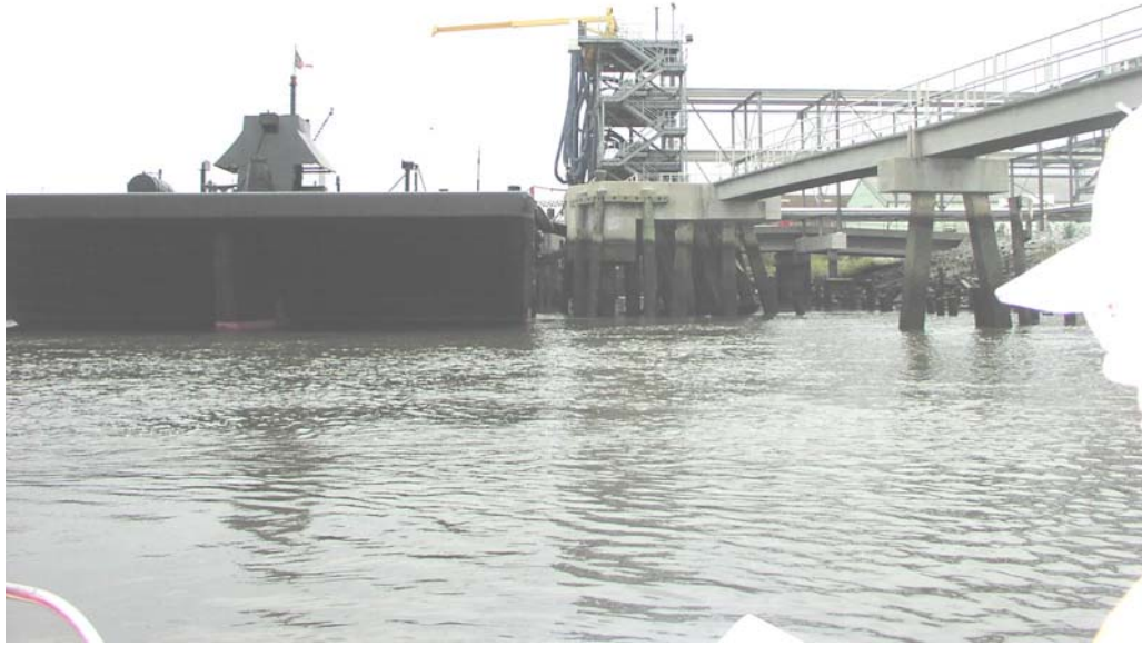
Colonial Terminals, Approx. Station 83+000, Piling in Good Condition
