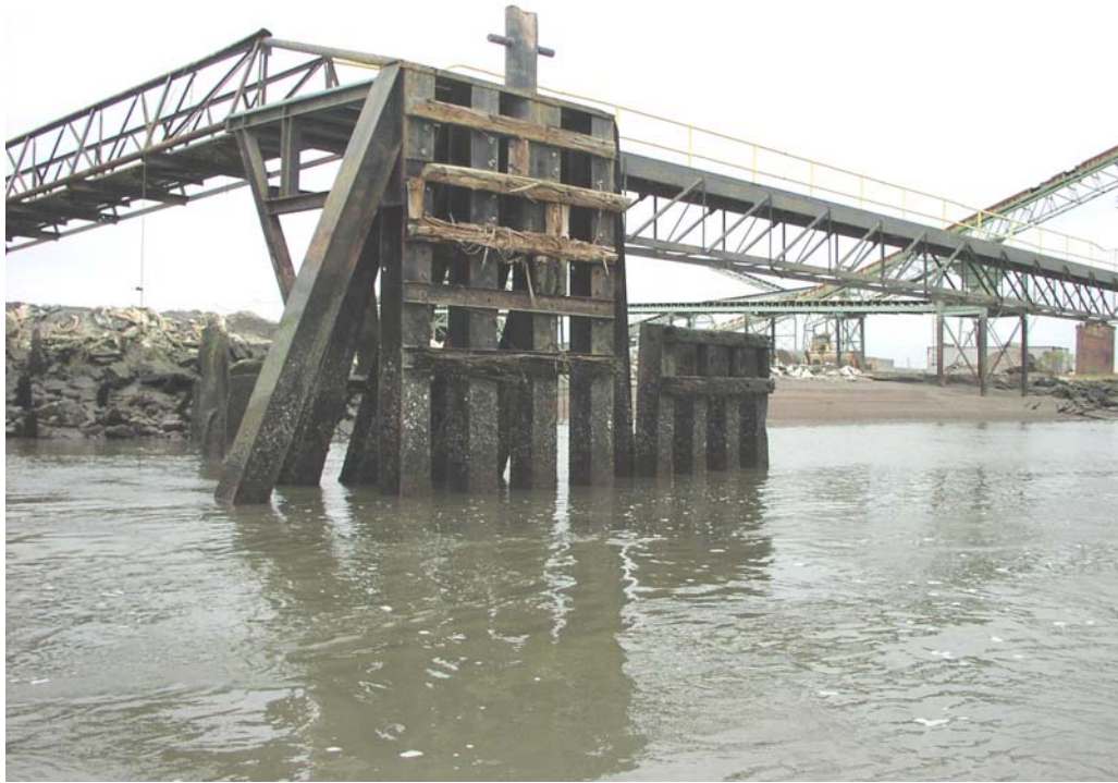
Wood Chip Facility, Station 66+800, Steel Piling, Good Condition
