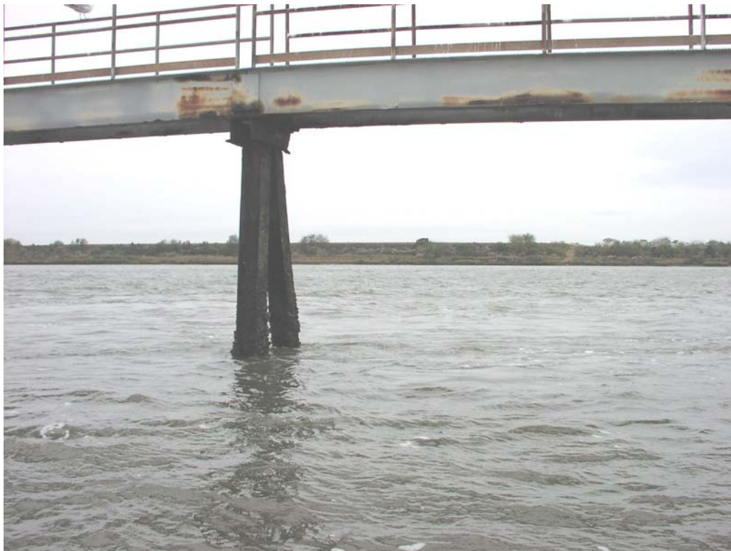
Kemira Inc. Dock and Pier. Stations 57+000 to 58+000, Piling Foundation – Good Condition, Steel Dock Beams Showing Deterioration
