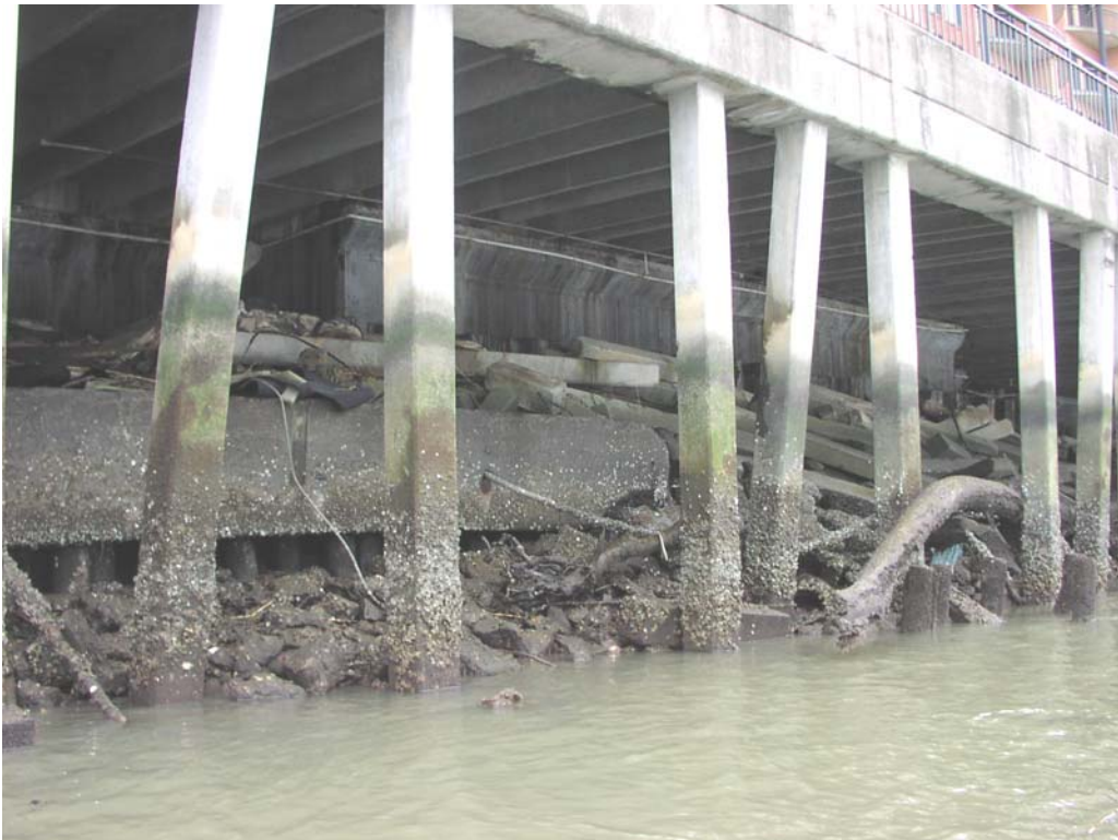
Marriott Hotel, Concrete Piles, Station 72+350, Good Condition
