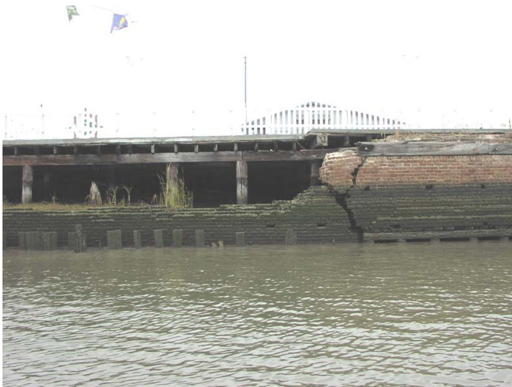
Crescent Towing & Salvage Company, Station 75+600, Brick Retaining Wall
