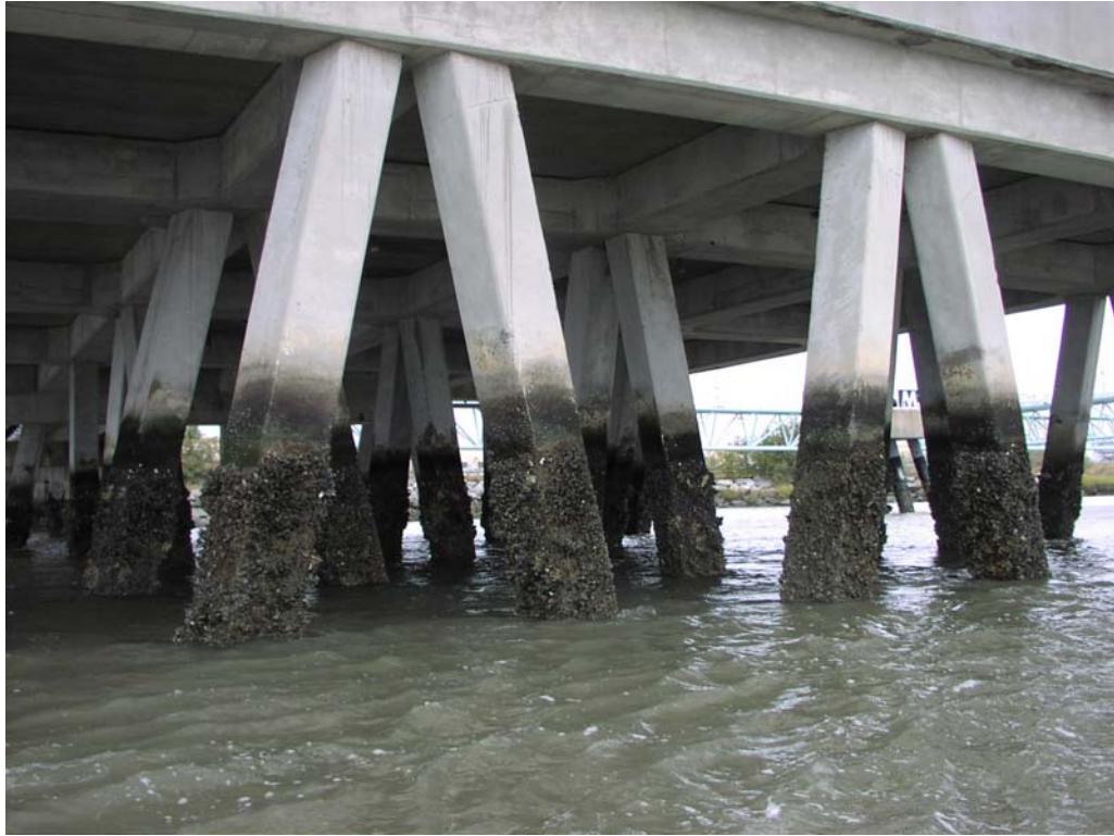
Southern Energy Company LNG–Dock Piling between Stations 38+300 to 39+500, Concrete Piling, Excellent Condition
