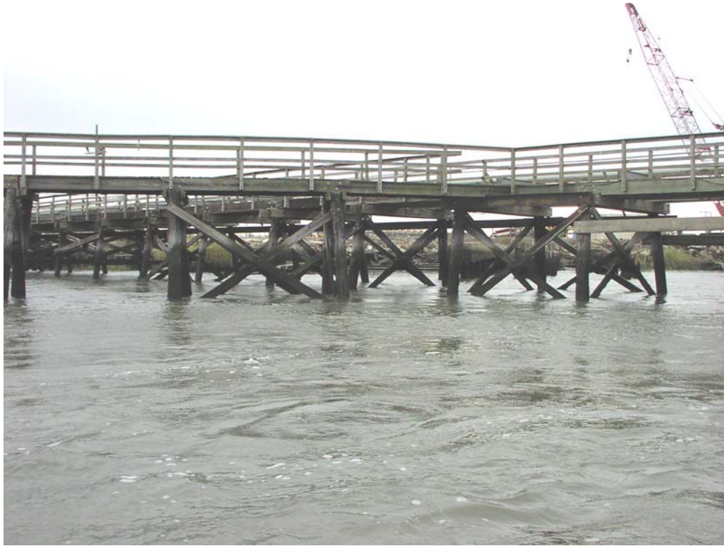
Unocal, Station 61+800, Wood Piling, Good Condition
