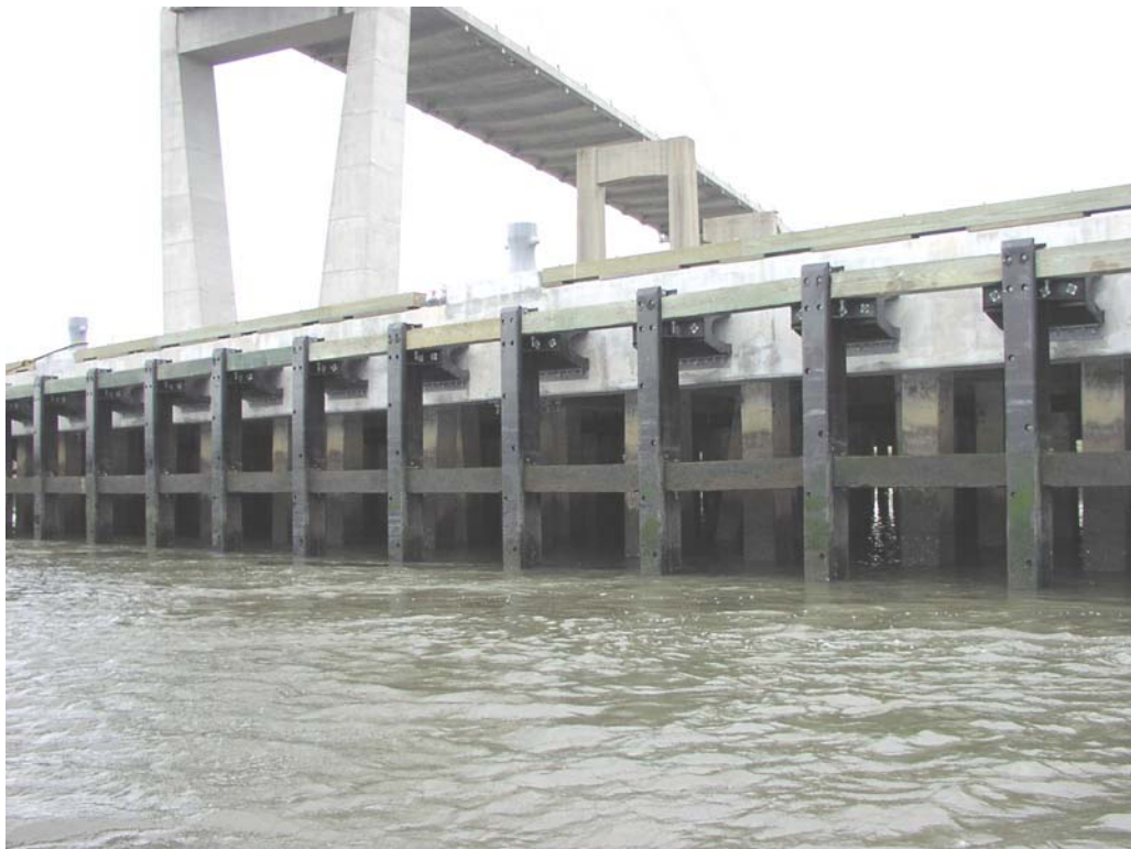
Georgia Ports Authority Berth 13, Station 79+700, Concrete Piles, Excellent Condition
