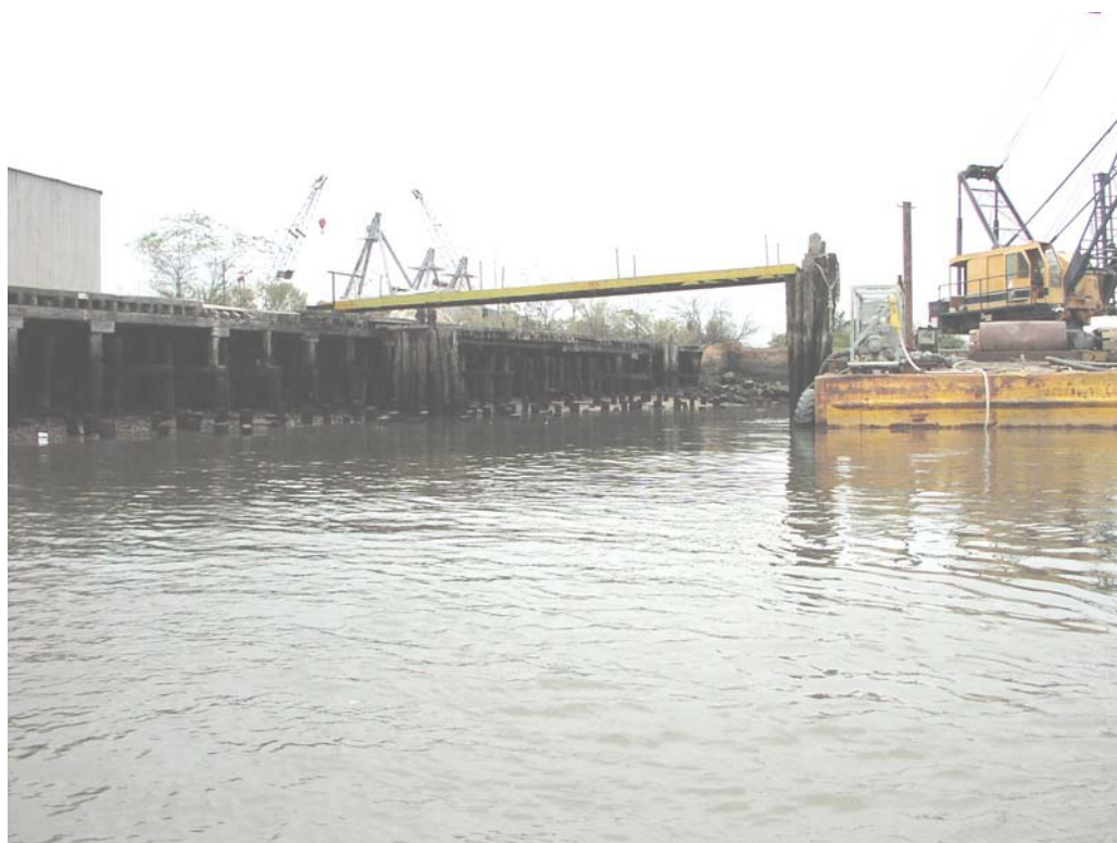
East Coast Terminal, Station 70+000, Wood Piling, Deteriorated Condition
