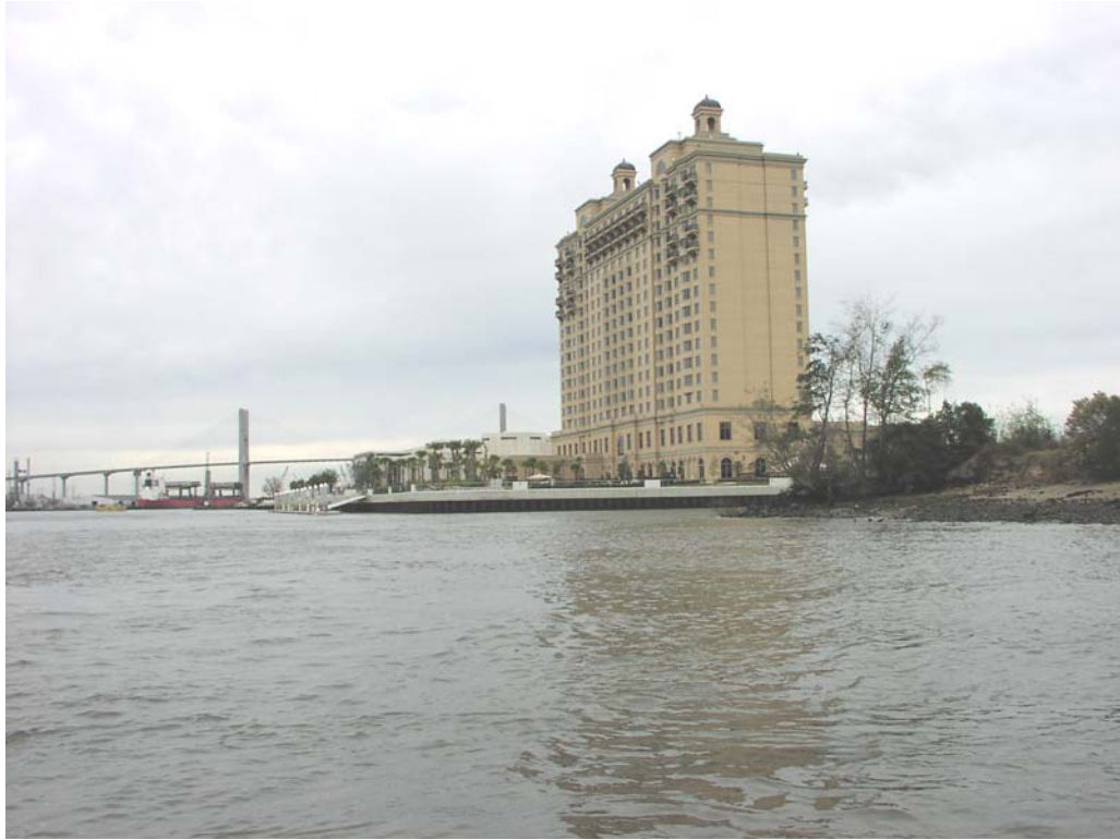
Weston Hotel, Steel Sheet Piles, Station 74+000, Good Condition
