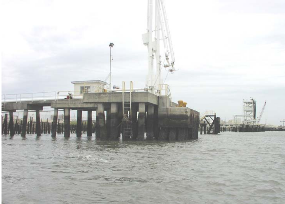
Unocal, Concrete Piles, Station 61+000, Good Condition
