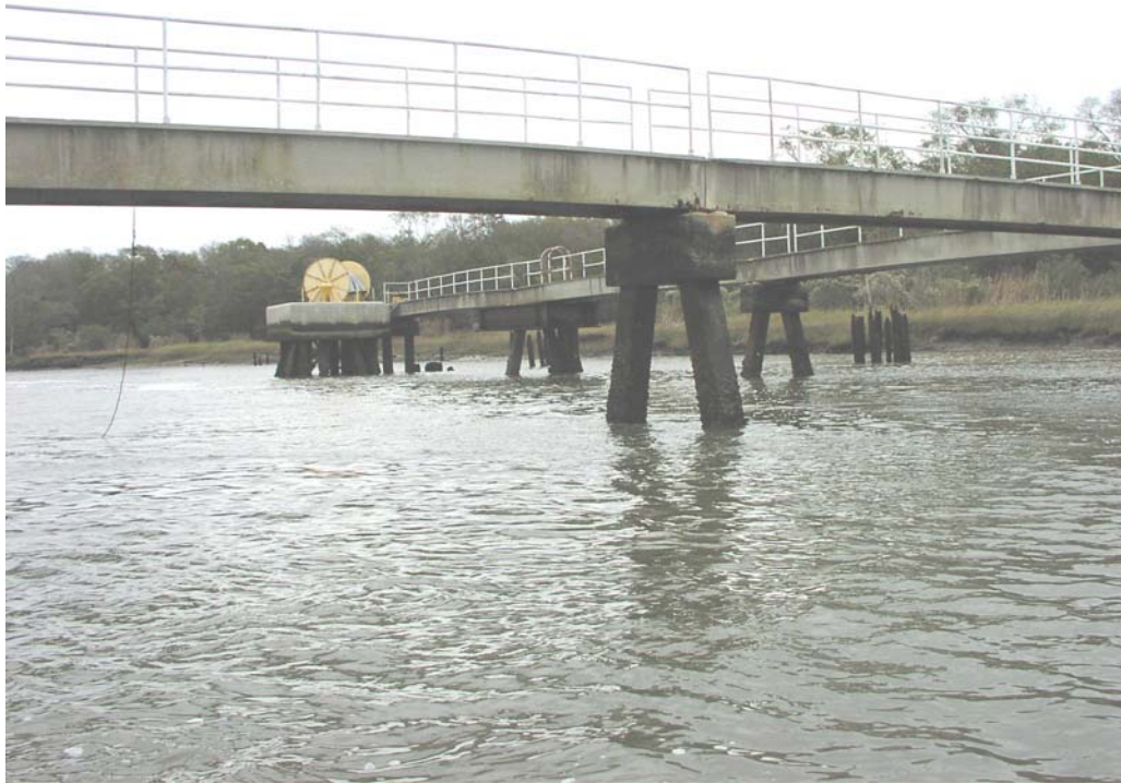
ST Services #1, Concrete Piling, Station 60+500, Good Condition
