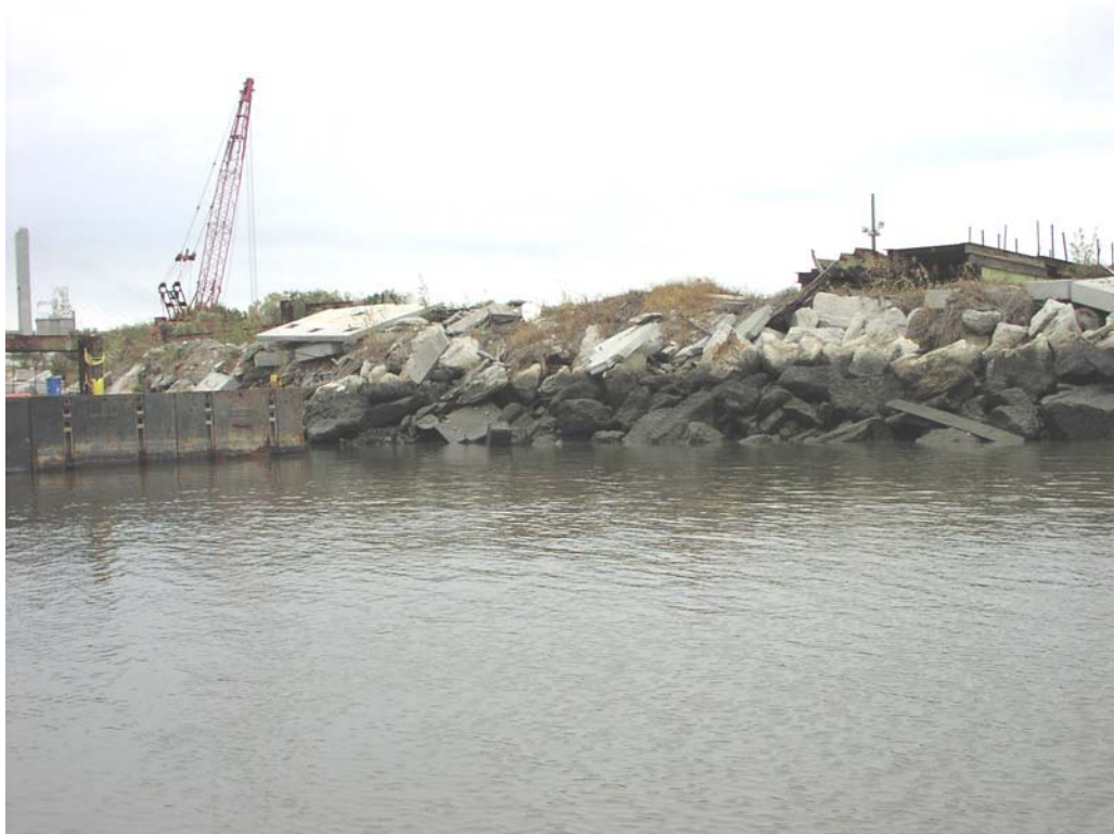
TIC, Station 76+000, Spud Barge
