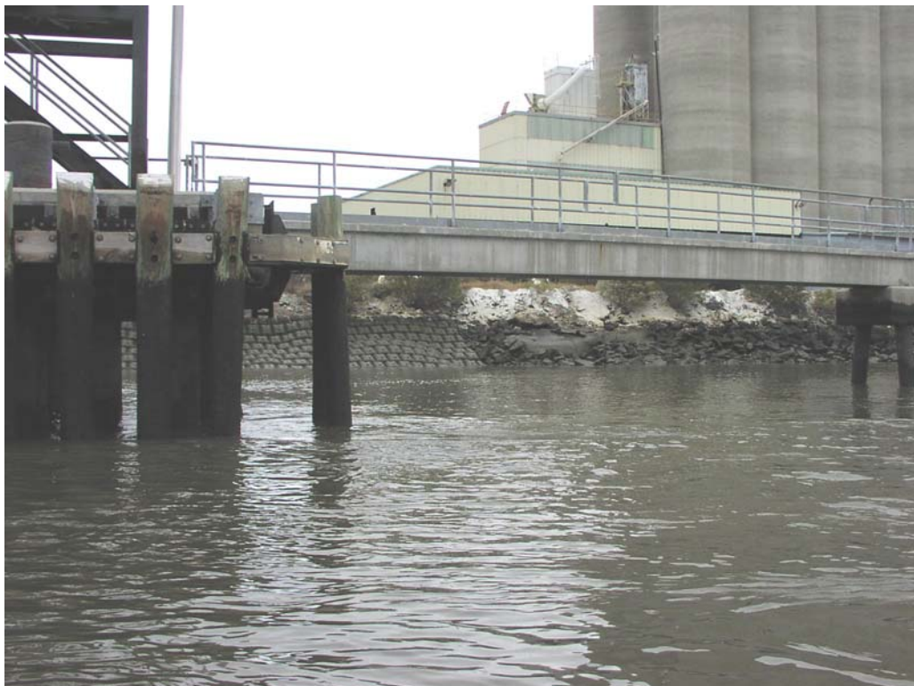
Blue Circle Cement, Approx. Station 78+800, Steel Shell Piles, Excellent Condition
