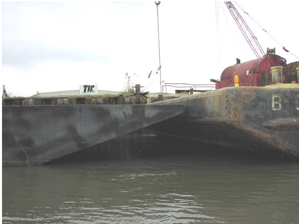
TIC, Approx. Station 76+100, Steel Sheet Piling in Good Condition
