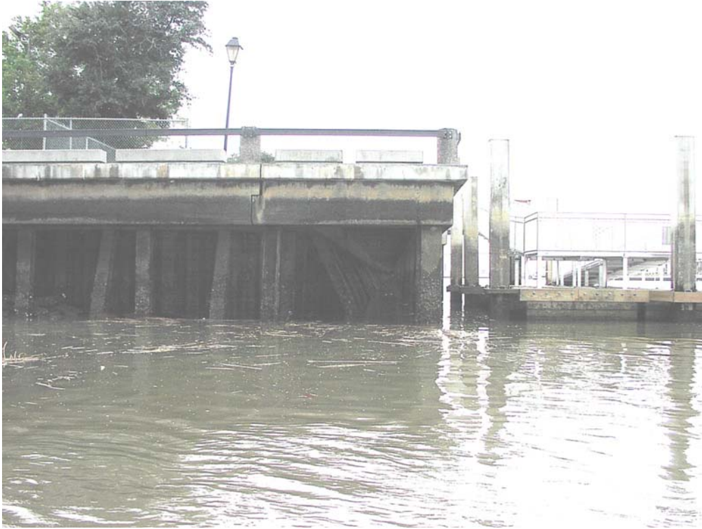
River Walk/Savannah Electric, Concrete Piles, Station 72+600, Good Condition
