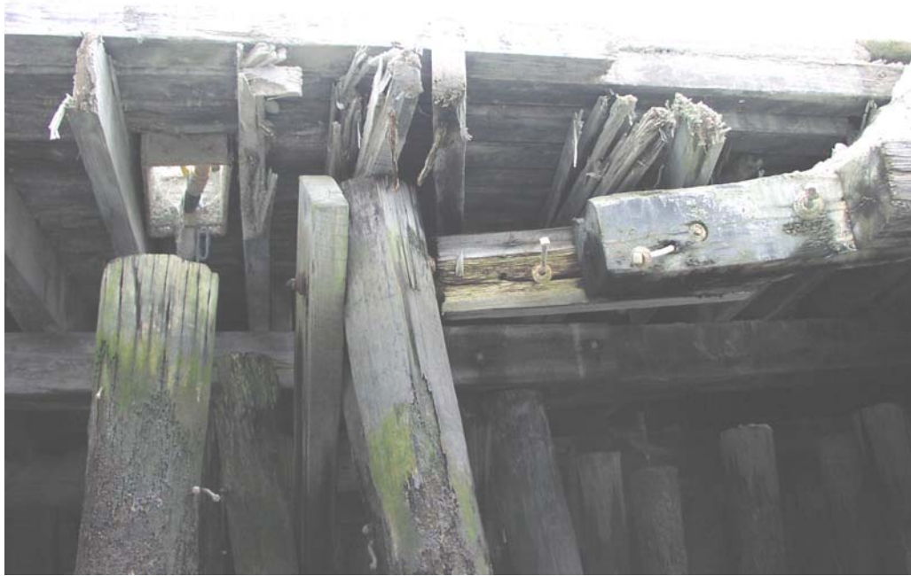
East Coast Terminal, Station 68+100, Wood Piling, Berth 4, Deteriorated/Broken Condition
