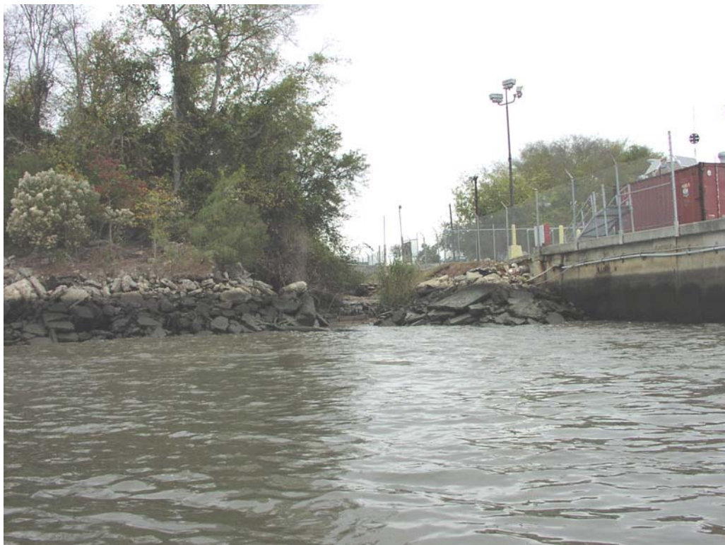
U.S. Army Corps of Engineers Yard, Concrete Sheet Piles, Station 72+800, Good Condition
