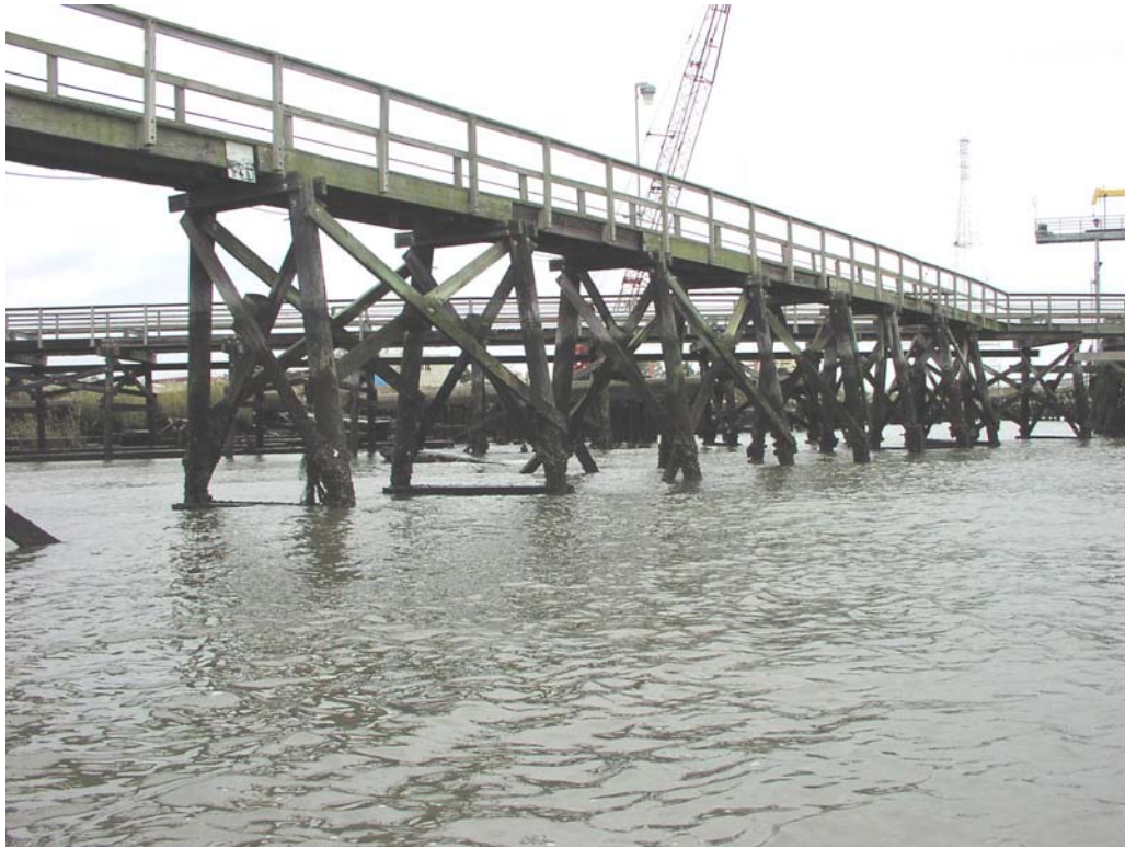
ST Services #2, Station 61+900, Wood Piles, Fair Condition
