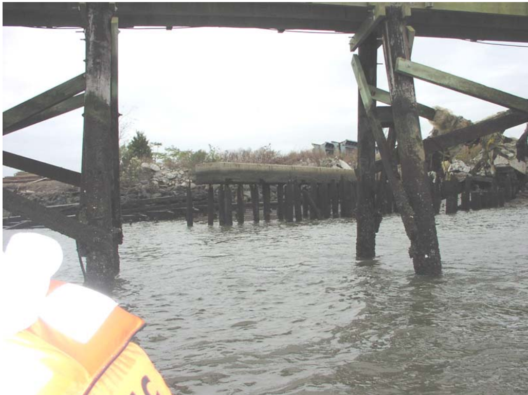
ST Services #2, Station 62+300, Wood Piles, Fair Condition
