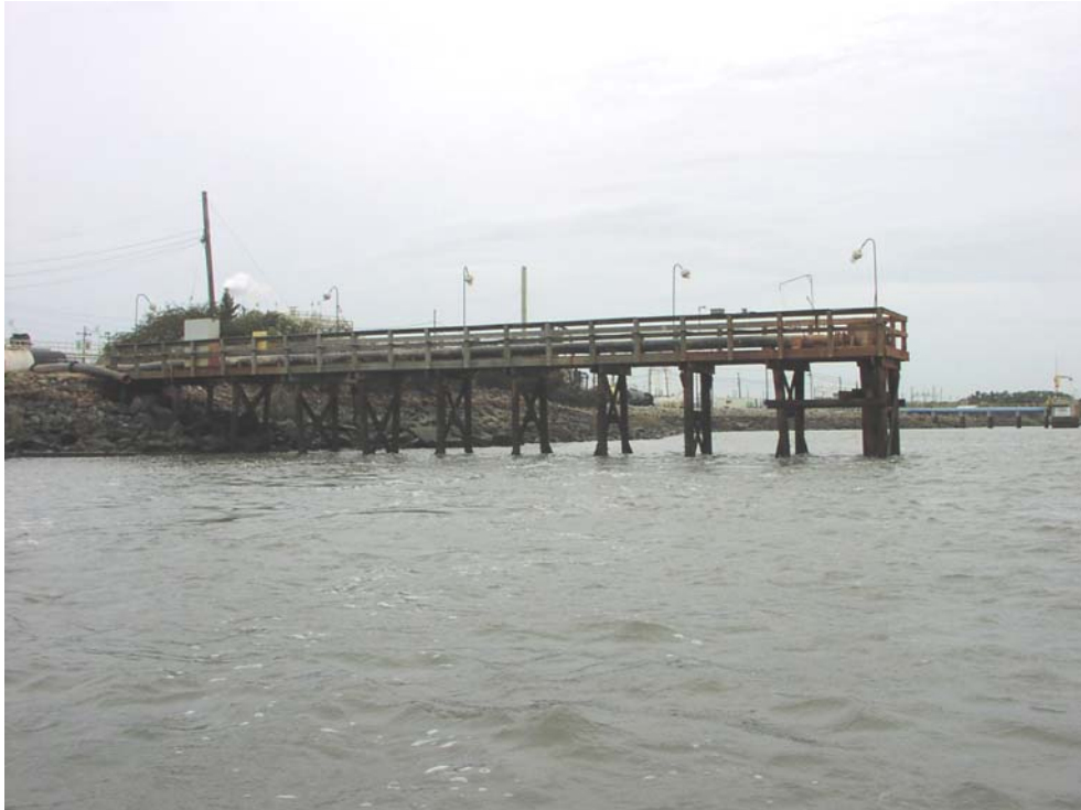
Kemira Inc. River Station 56+000, Pipe Dock. Wood Piles, Good Condition
