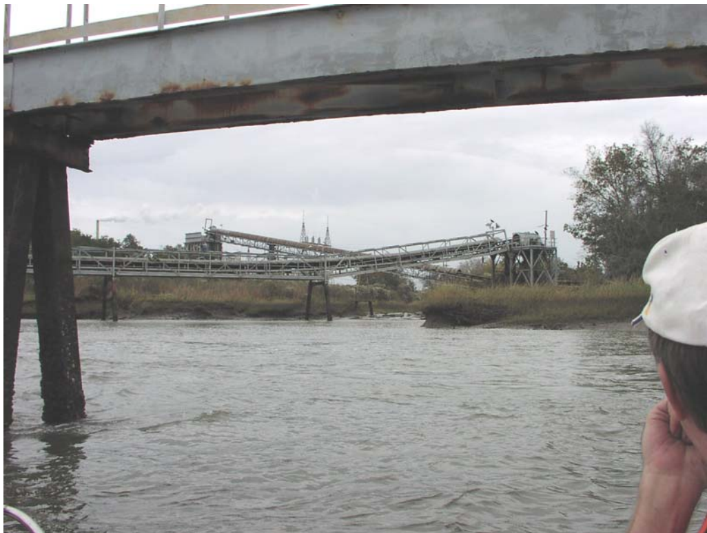
Kemira Inc. Dock and Pier. Stations 57+000 to 58+000, Piling Foundation – Good Condition,
