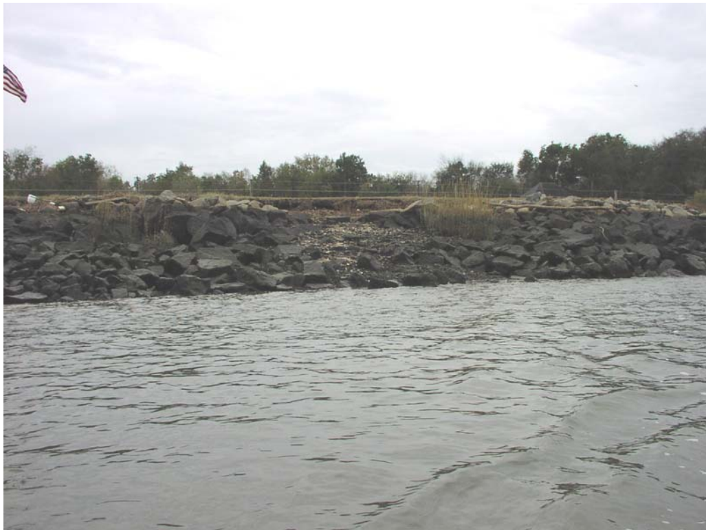
Old Fort Jackson, Upstream Riprap, Station 58+700
