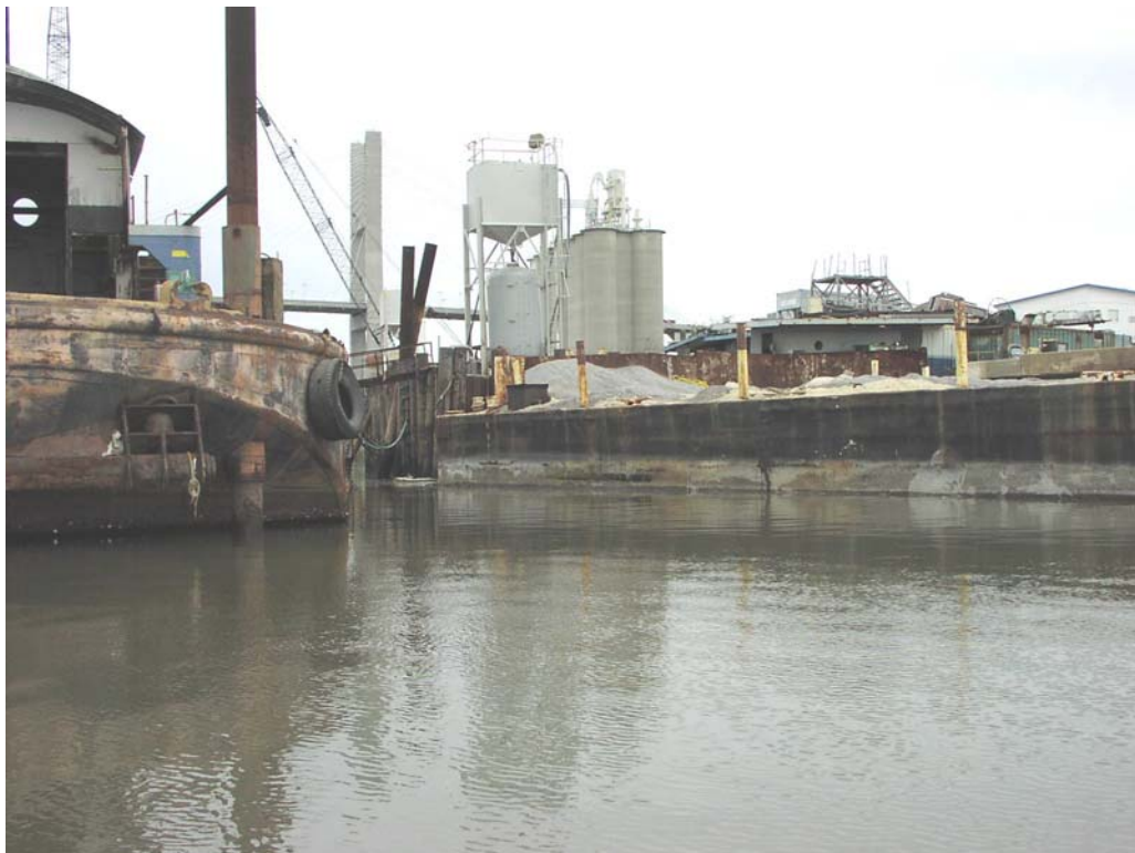
Savannah Marine Services, Station 77+250
