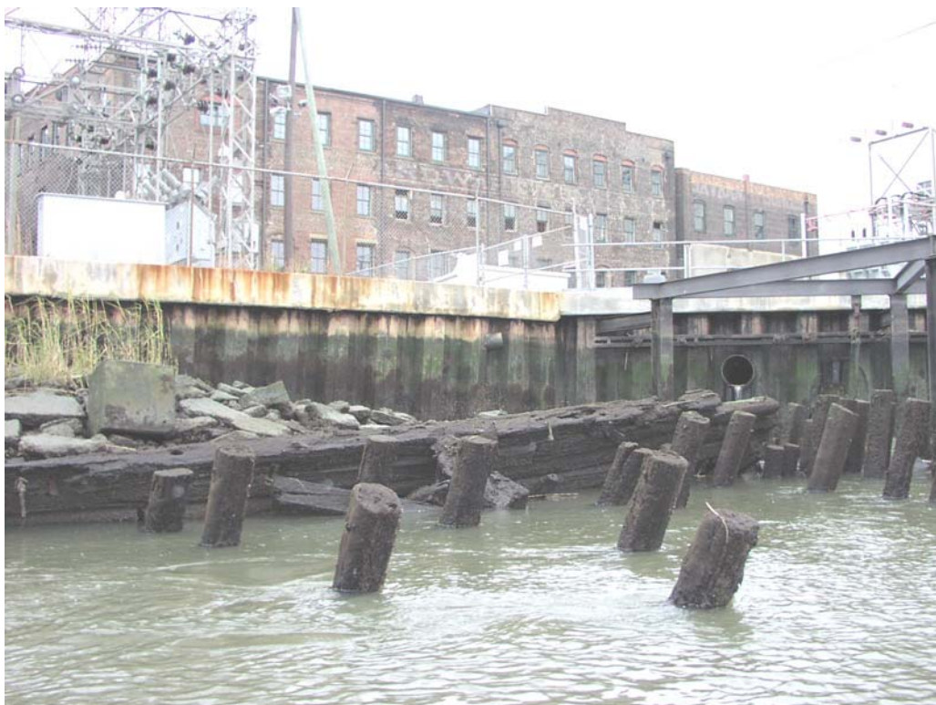
River Street/Savannah Electric, Station 77+000
