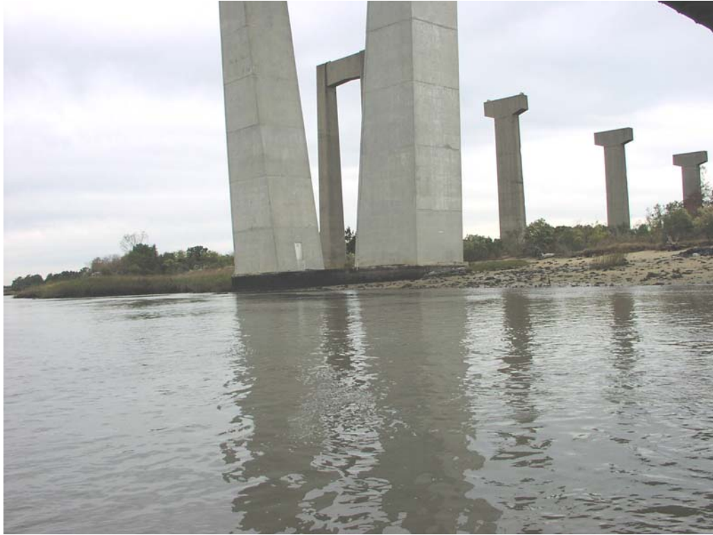
Tallmadge Bridge Pier North Side, Station 79+300, Good Condition
