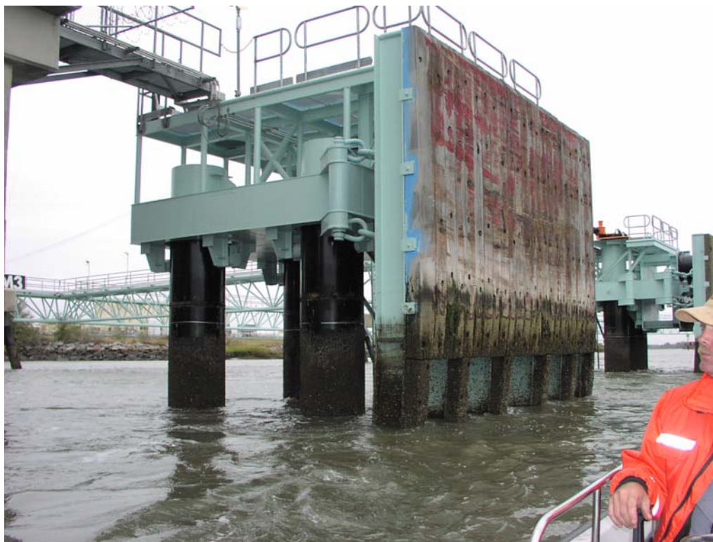
Southern Energy Company LNG–Dock Fender between Stations 38+300 to 39+500, Steel Piling, Excellent Condition
