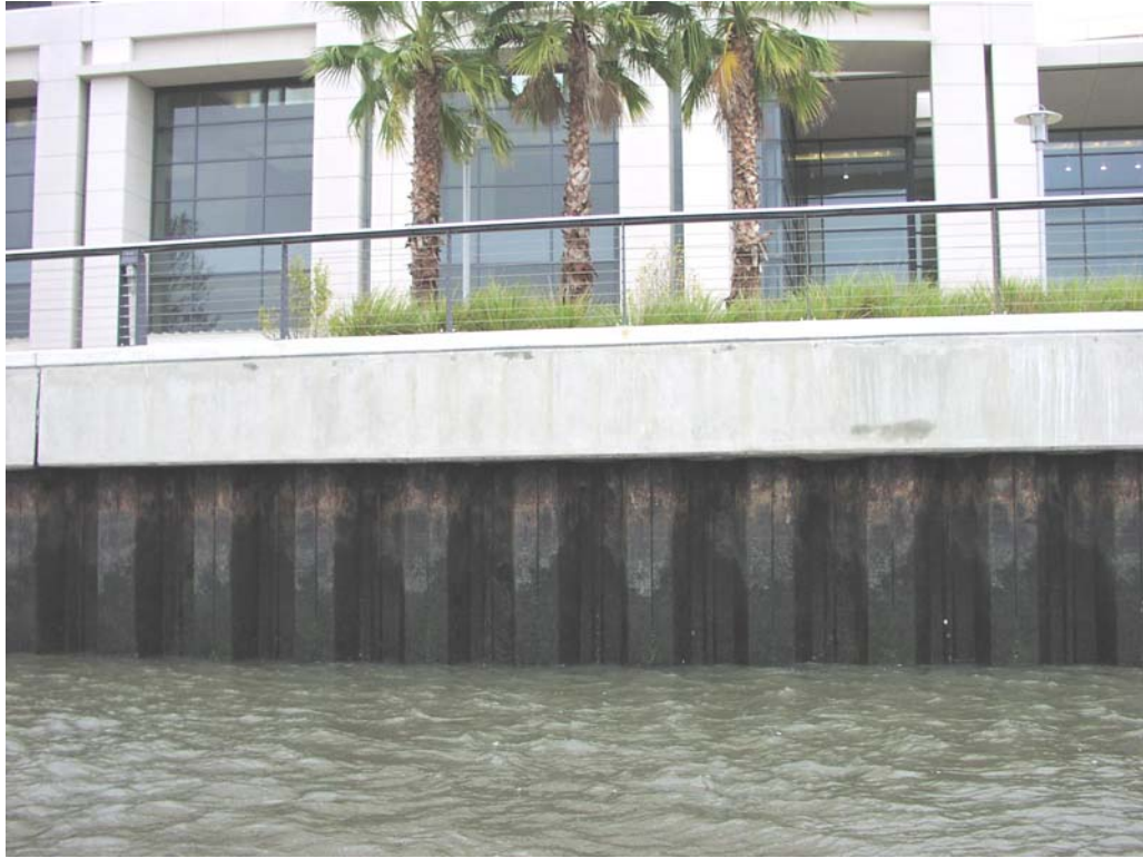
Convention Center, Steel Sheet Piles, Station 74+700, Good Condition
