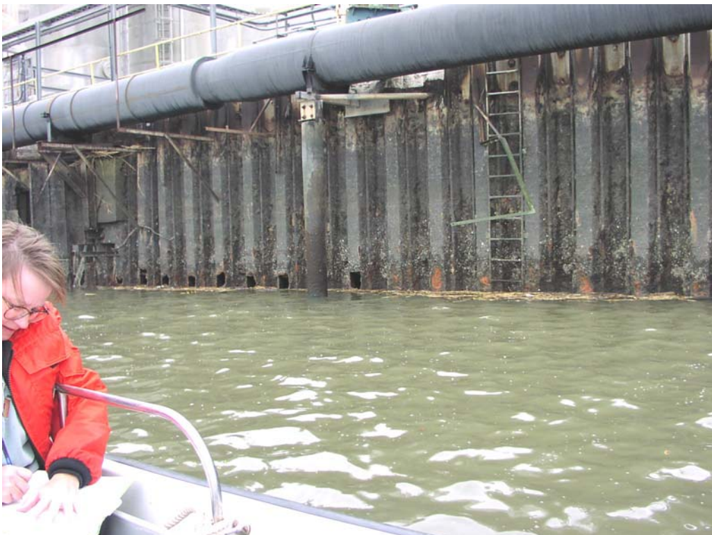
Union Camp Corp., Approx. Station 88+000, Steel Sheet Piling rusted thru at low water line
