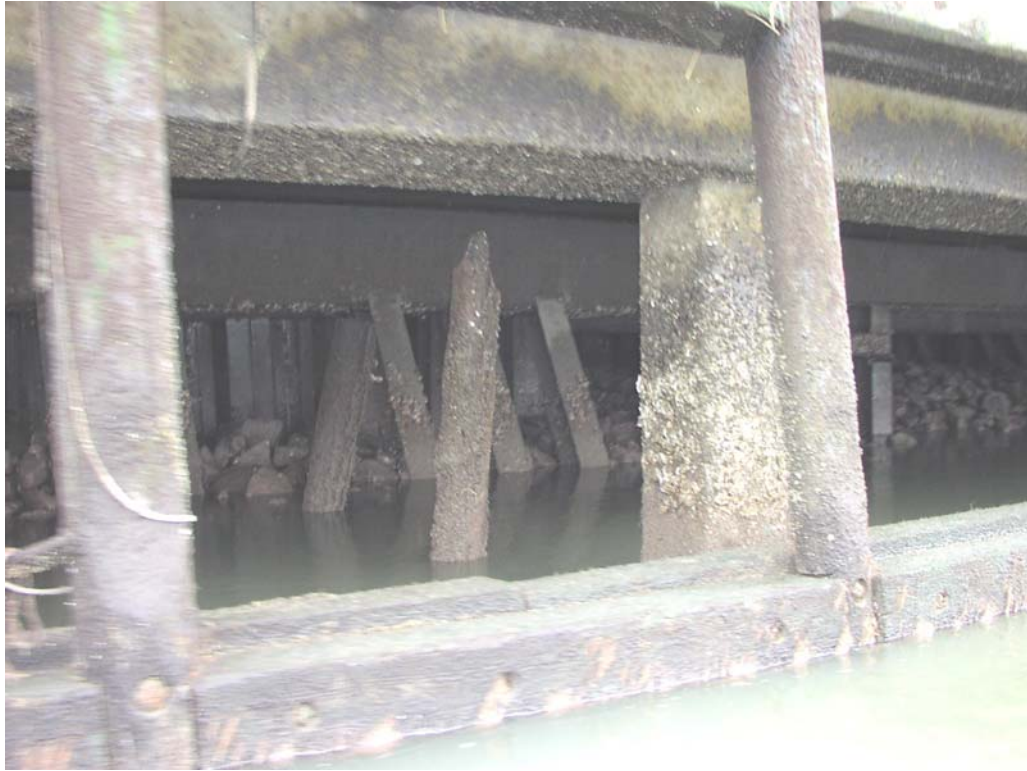
River Street, Approximate Station 75+500, Hyatt Area
