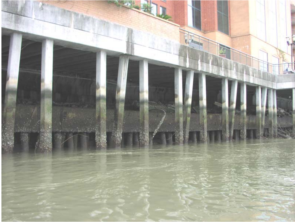
Marriott Hotel, Concrete Piles, Station 72+300, Good Condition
