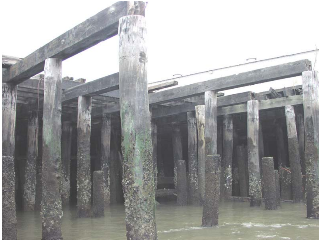
East Coast Terminal, Station 69+400, Wood Piling, Deteriorated/Broken Condition
