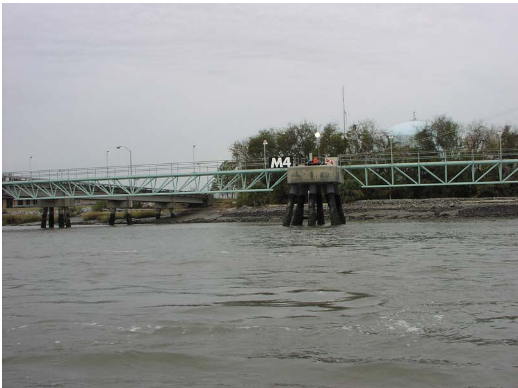
Southern Energy Company LNG–Location M2 between Stations 38+300 to 39+500, Concrete and Steel Piling, Excellent Condition
