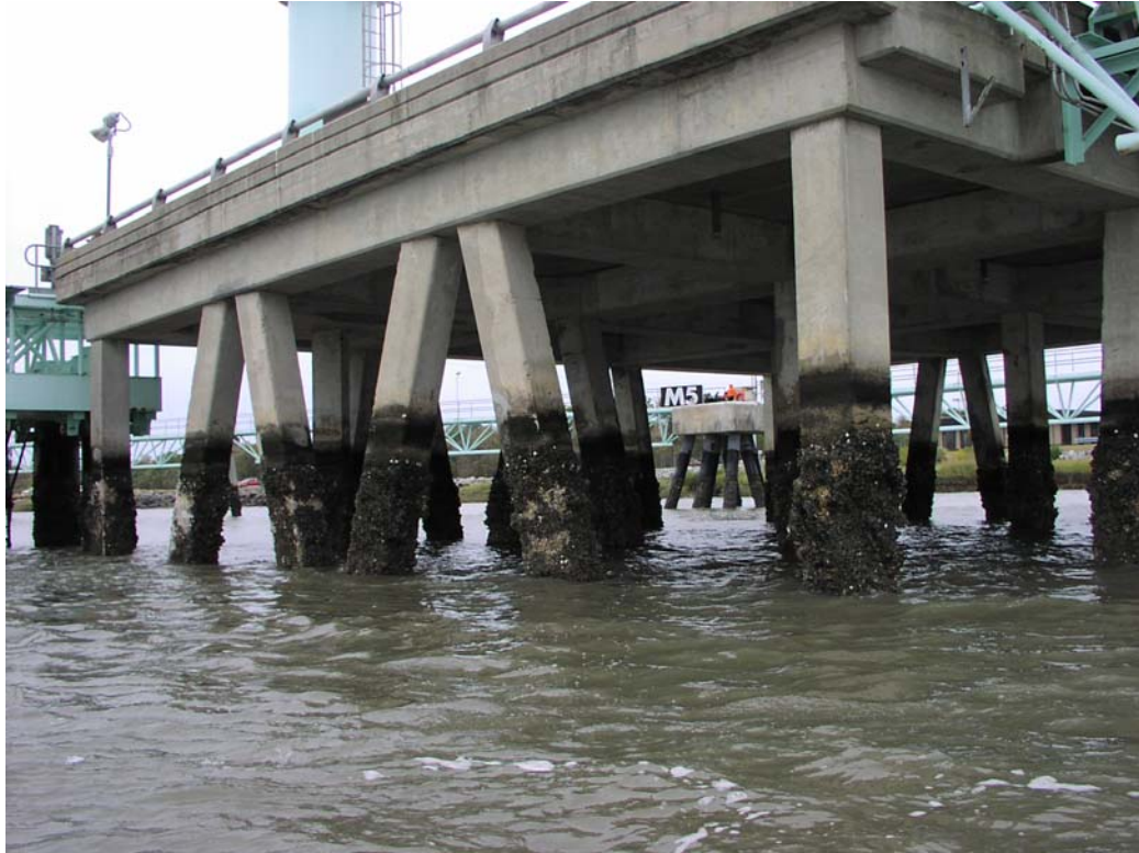
Southern Energy Company LNG–Dock and Piling between Stations 38+300 to 39+500, Concrete Piling, Excellent Condition
