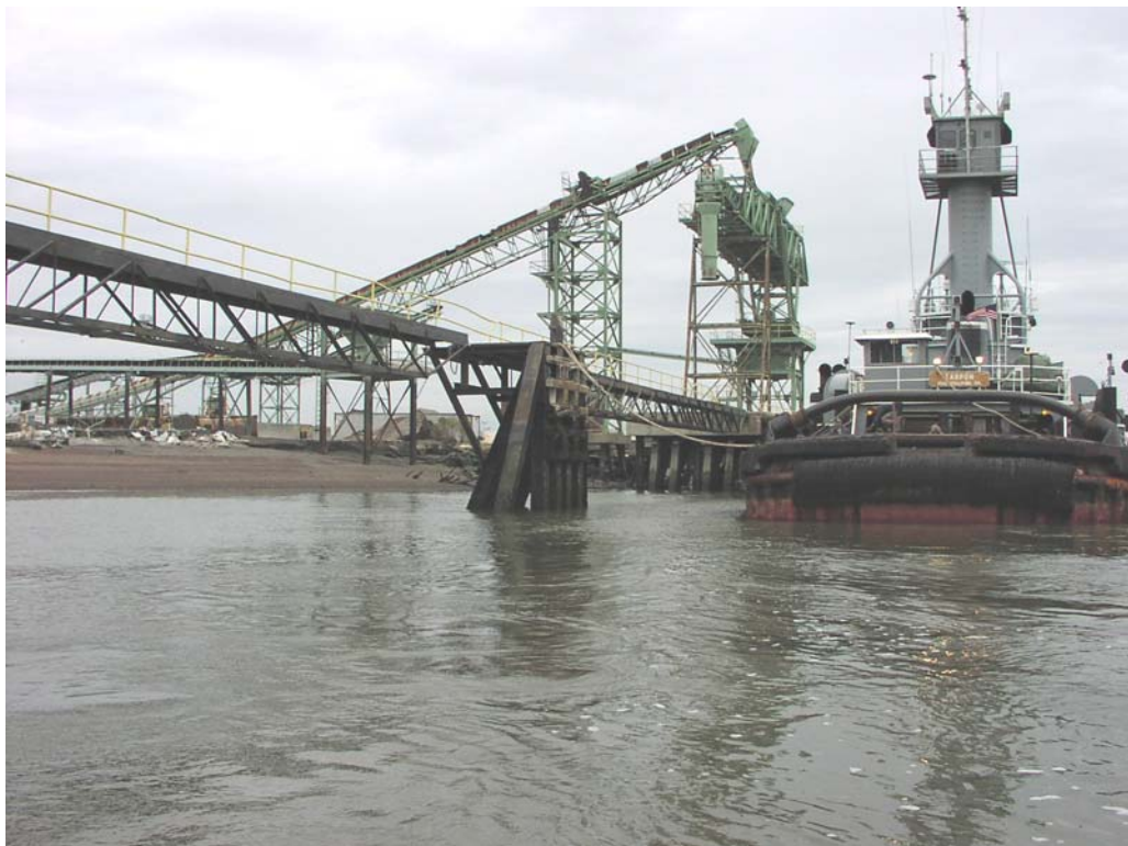
Wood Chip Facility, Station 67+000, Steel Piling, Good Condition
