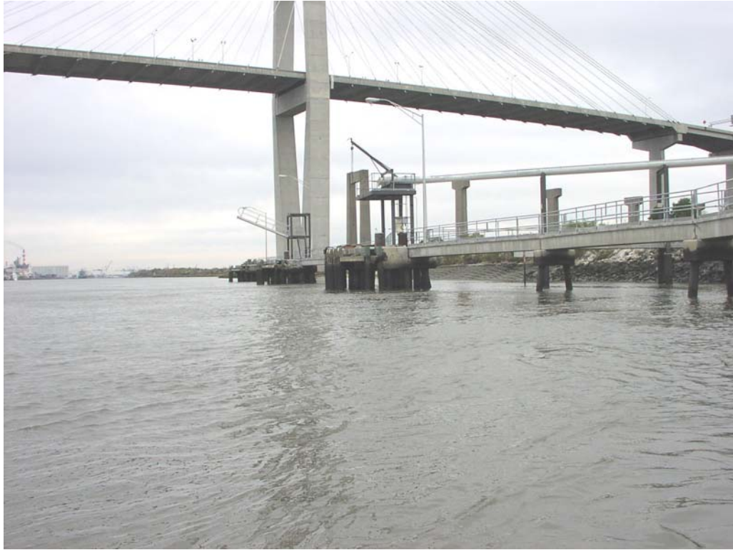
Blue Circle Cement, Approx. Station 78+600, Steel Shell Piles, Excellent Condition
