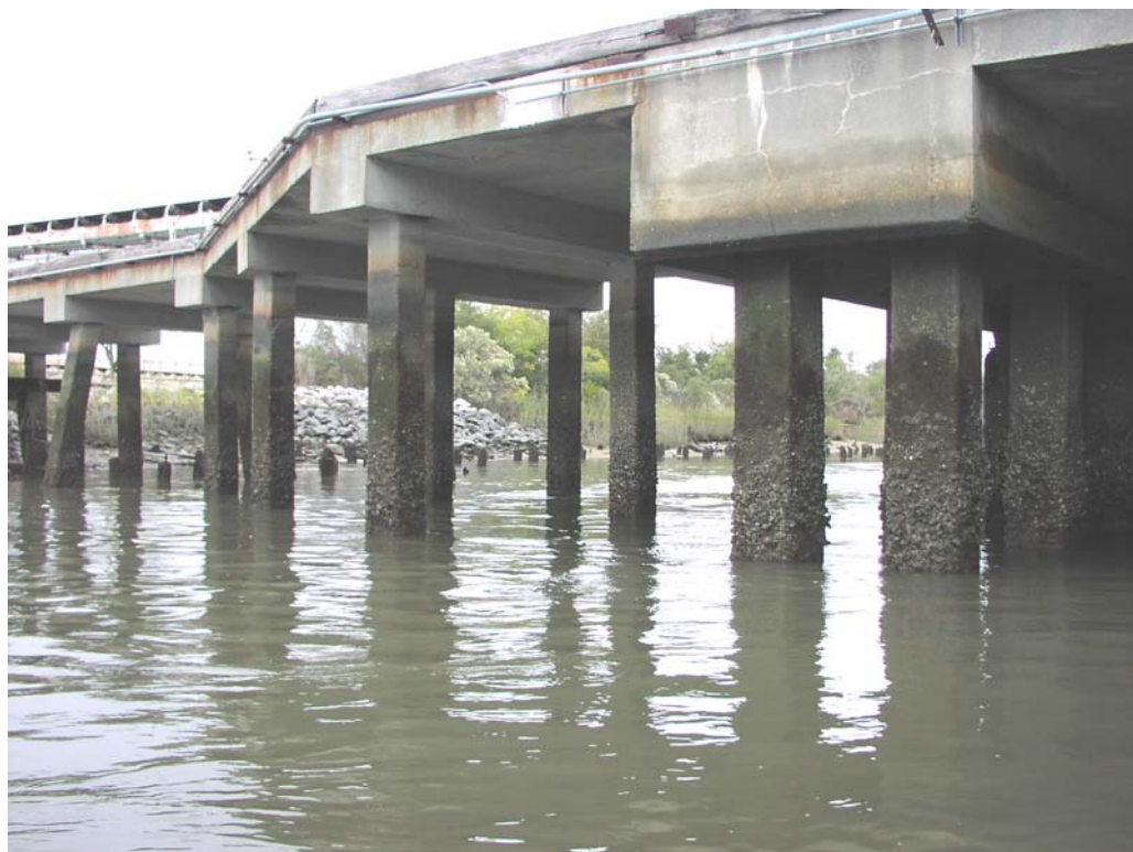
Georgia Pacific Gypsum, Station 63+250, Concrete Piles, Good Condition (Close-Up)
