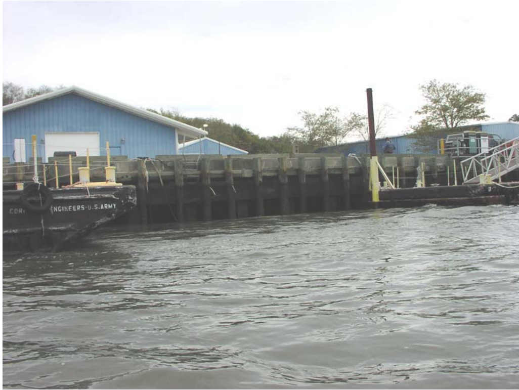
U.S. Army Corps of Engineers Yard, Concrete Piles, Station 72+500, Good Condition
