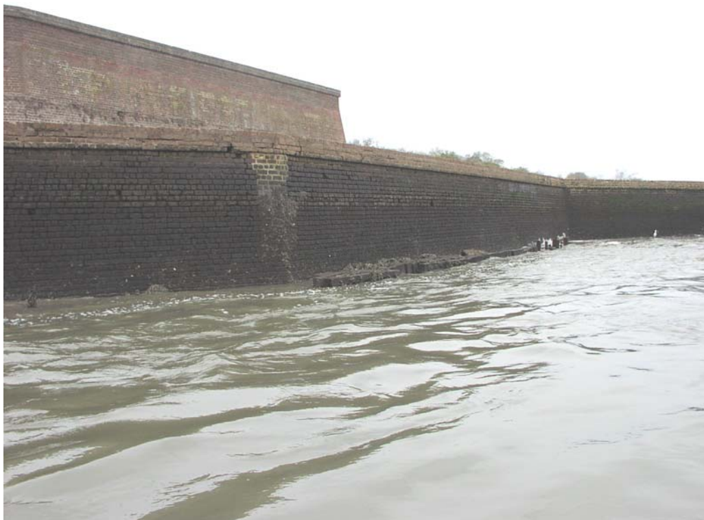
Old Fort Jackson, Downstream Moat Brickwork, Station 58+500
