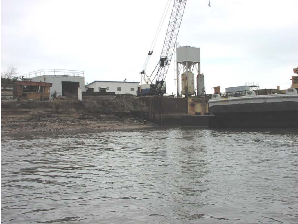
Savannah Marine Services, Station 77+350
