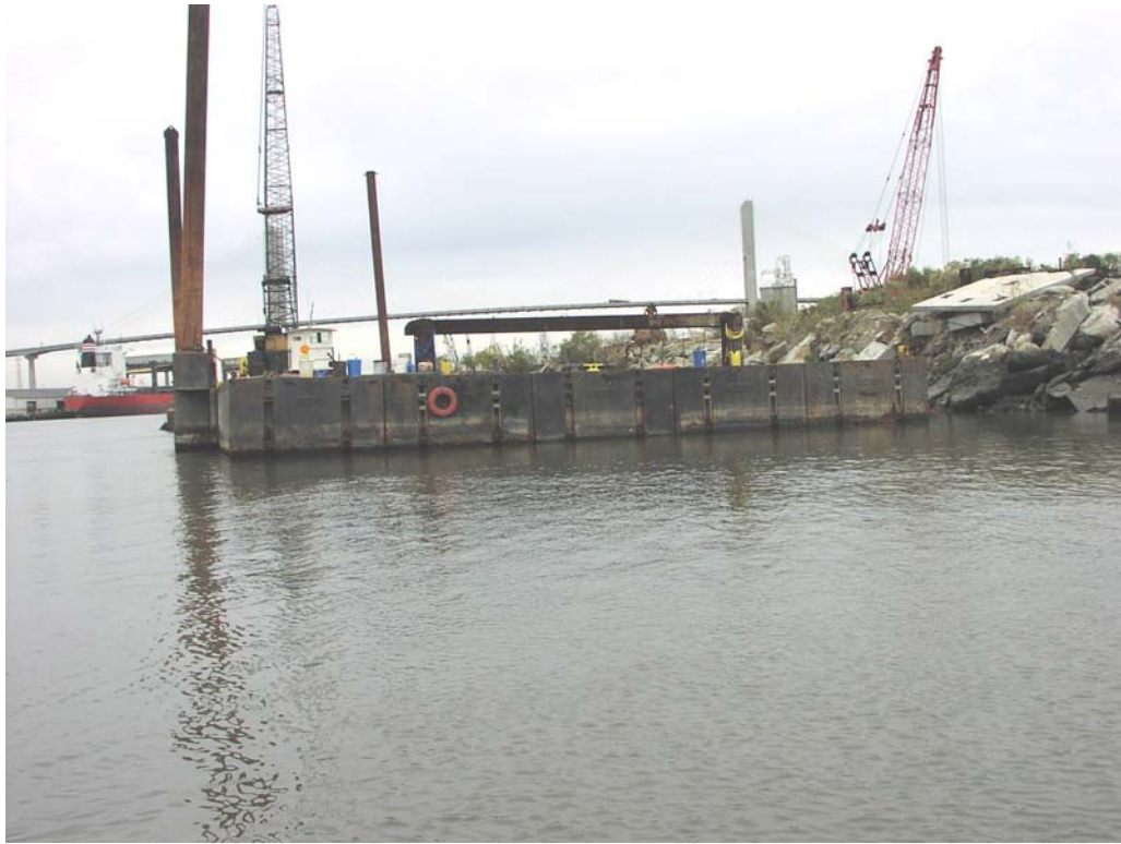
TIC, Station 76+000, Spud Barge
