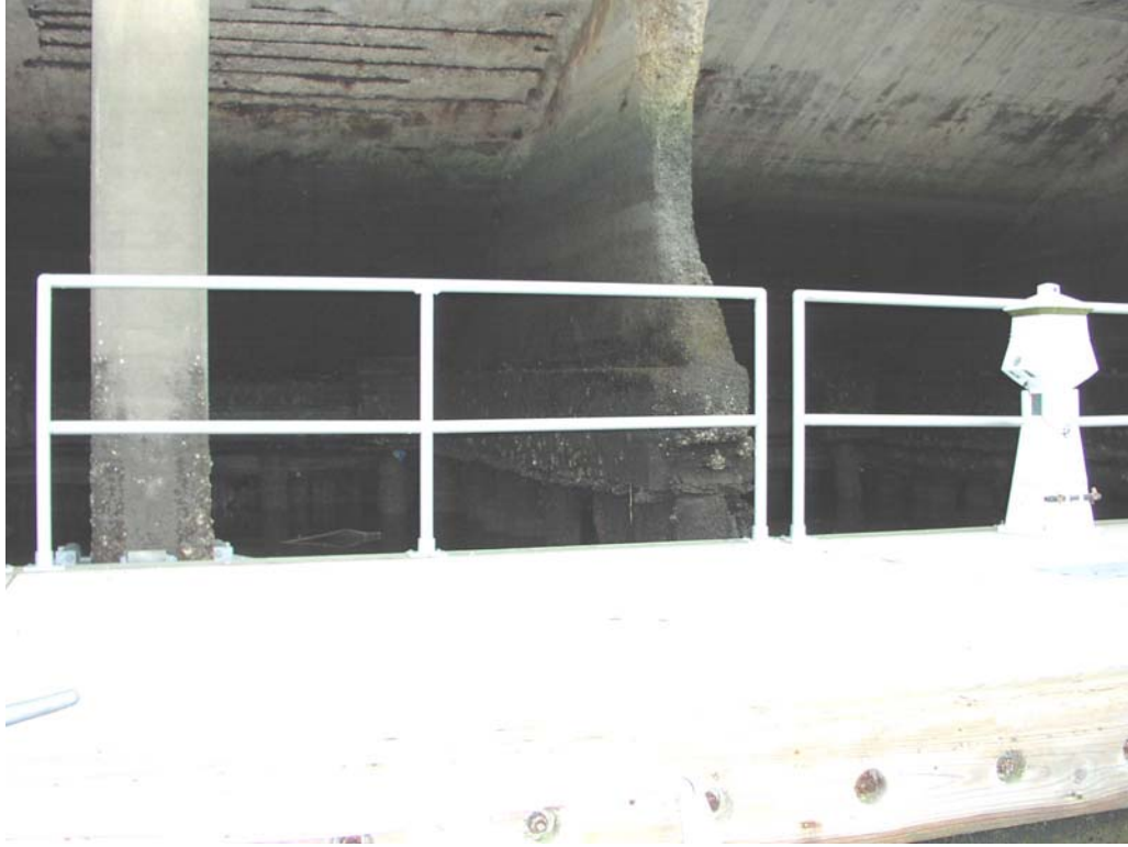
Turecamo/Parking Lot, Concrete Support on Wood Piles, Station 74+400, Poor Condition
