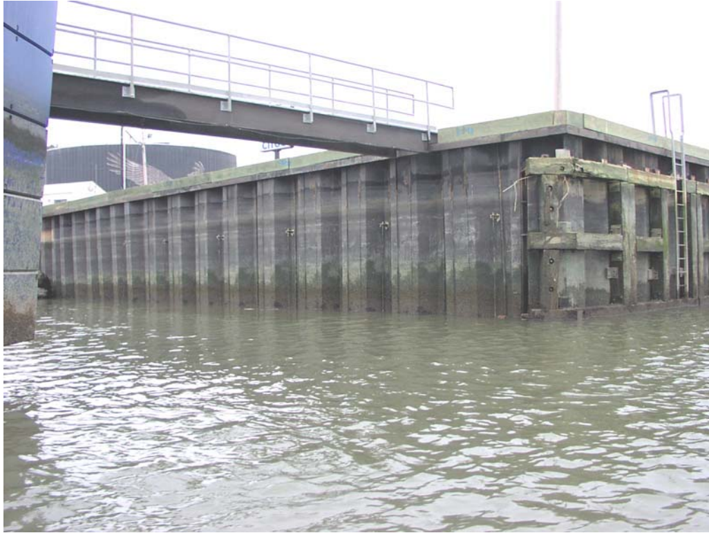
Union Camp Corp., Approx. Station 88+000, Steel Sheet Piling
