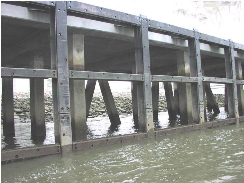
Citgo Asphalt Refining Co., Station 90+000, Steel Sheet Piling, Good Condition
