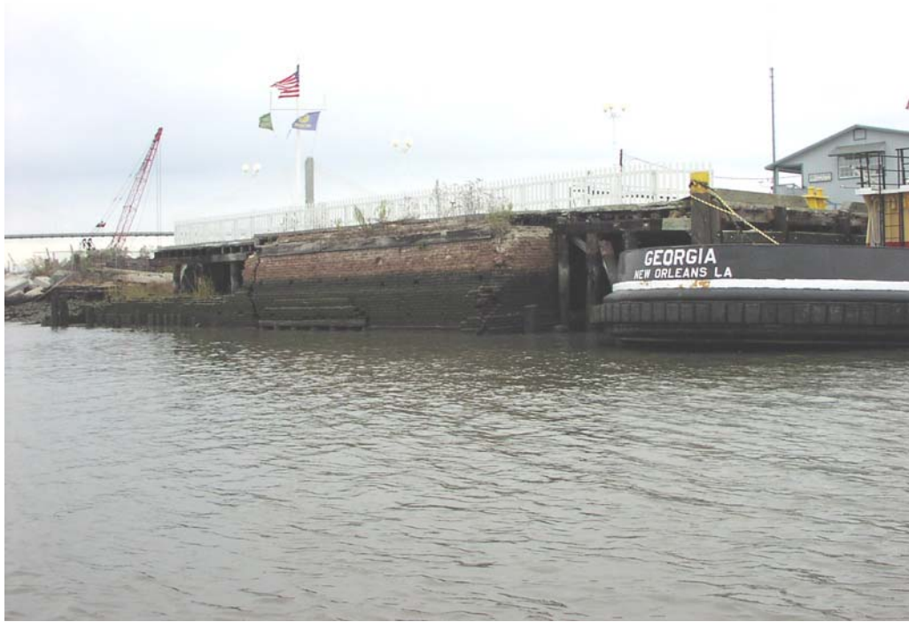
Crescent Towing & Salvage Company, Station 75+500, Brick Retaining Wall
