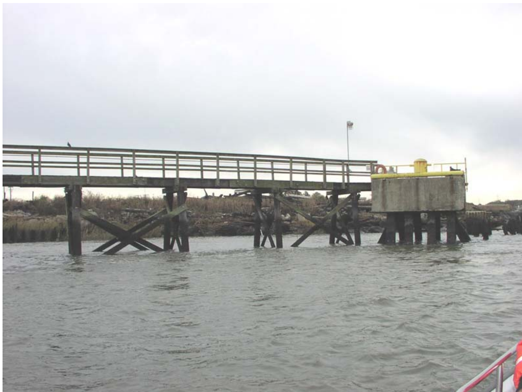
ST Services #2, Station 62+200, Wood/Steel Piling, Good Condition
