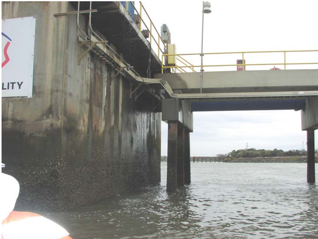
Kemira Inc. Dock and Pier. Stations 57+000 to 58+000, Foundation – Concrete and Steel, Good Condition
