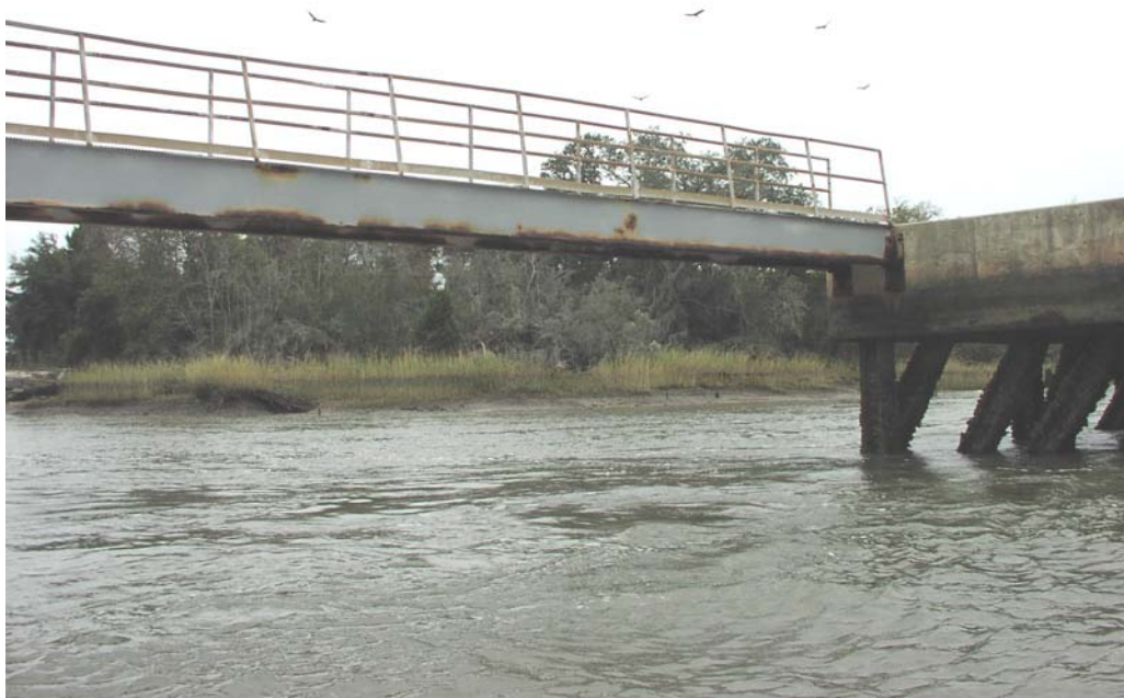
Kemira Inc. Dock and Pier. Stations 57+000 to 58+000, Piling Foundation – Good Condition, Steel Beams Showing Deterioration
