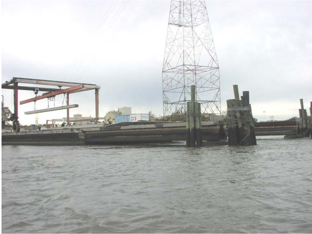
Standard Concrete Products, Station 62+600, Concrete Piers and Beams, Excellent Condition
