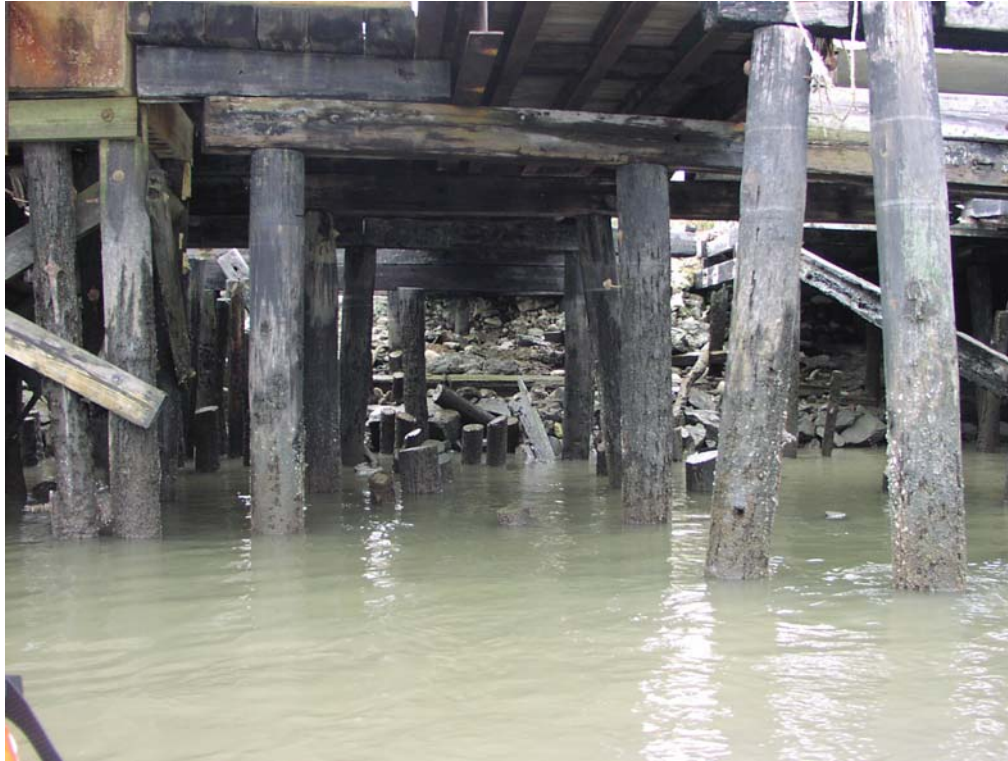
East Coast Terminal Company, Station 68+500, Wood Piles
