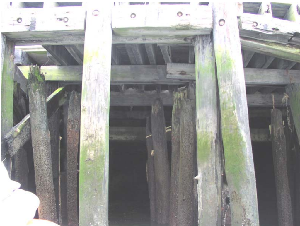
East Coast Terminal Company, Station 69+800, Wood Piles
