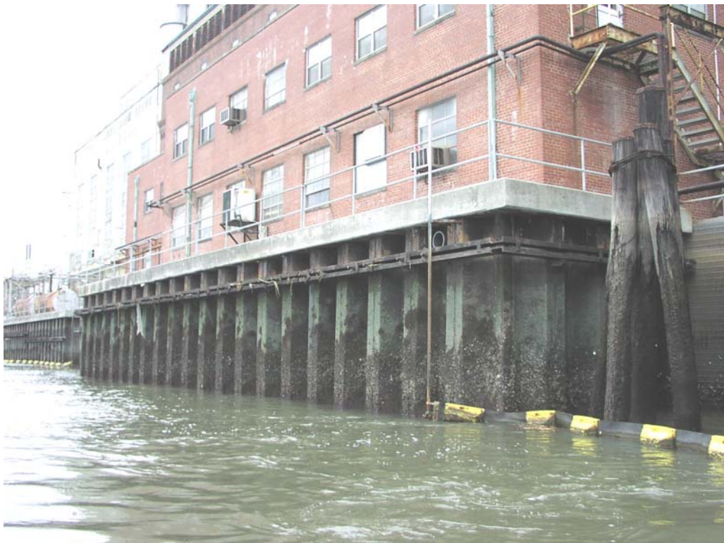
Savannah Electric Peaking Plant, Approx. Station 77+500, Good Condition
