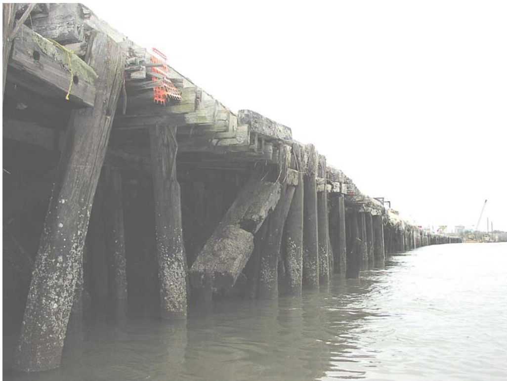
East Coast Terminal, Station 68+500, Wood Piling, Deteriorated/Broken Condition
