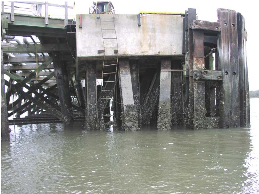
ST Services #2, Station 62+000, Steel Piles, Good Condition
