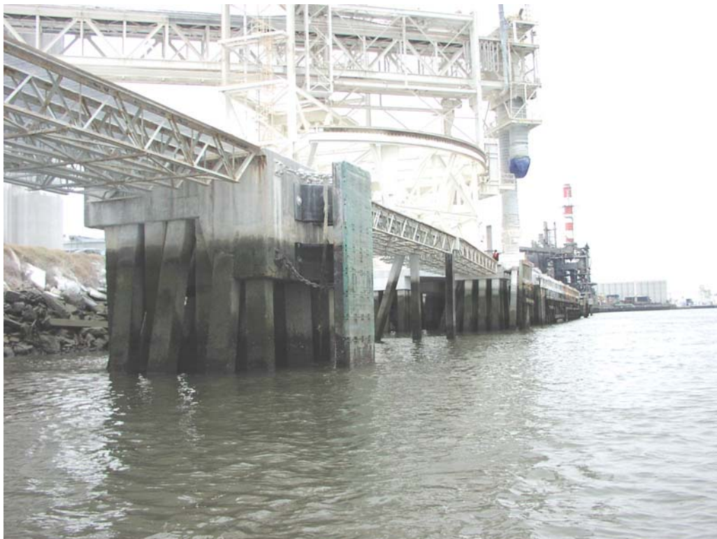
Colonial Terminals, Station 86+000, Concrete Piles, Excellent Condition
