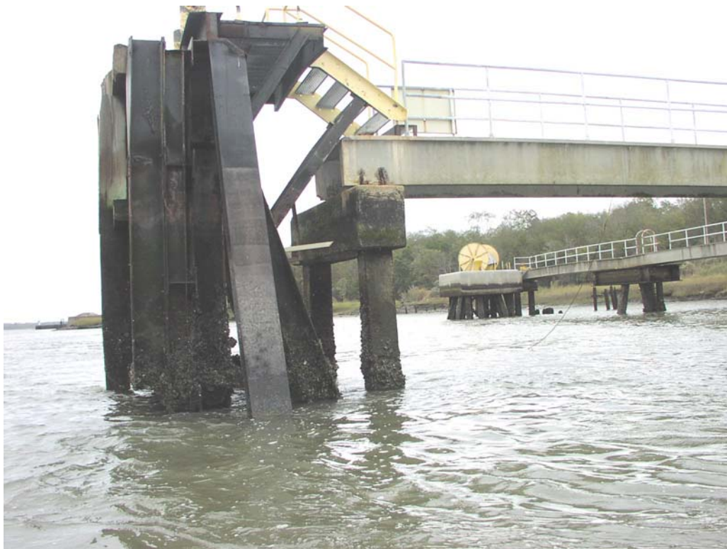
ST Services #1, Concrete and Steel Piling, Station 60+500, Good Condition
