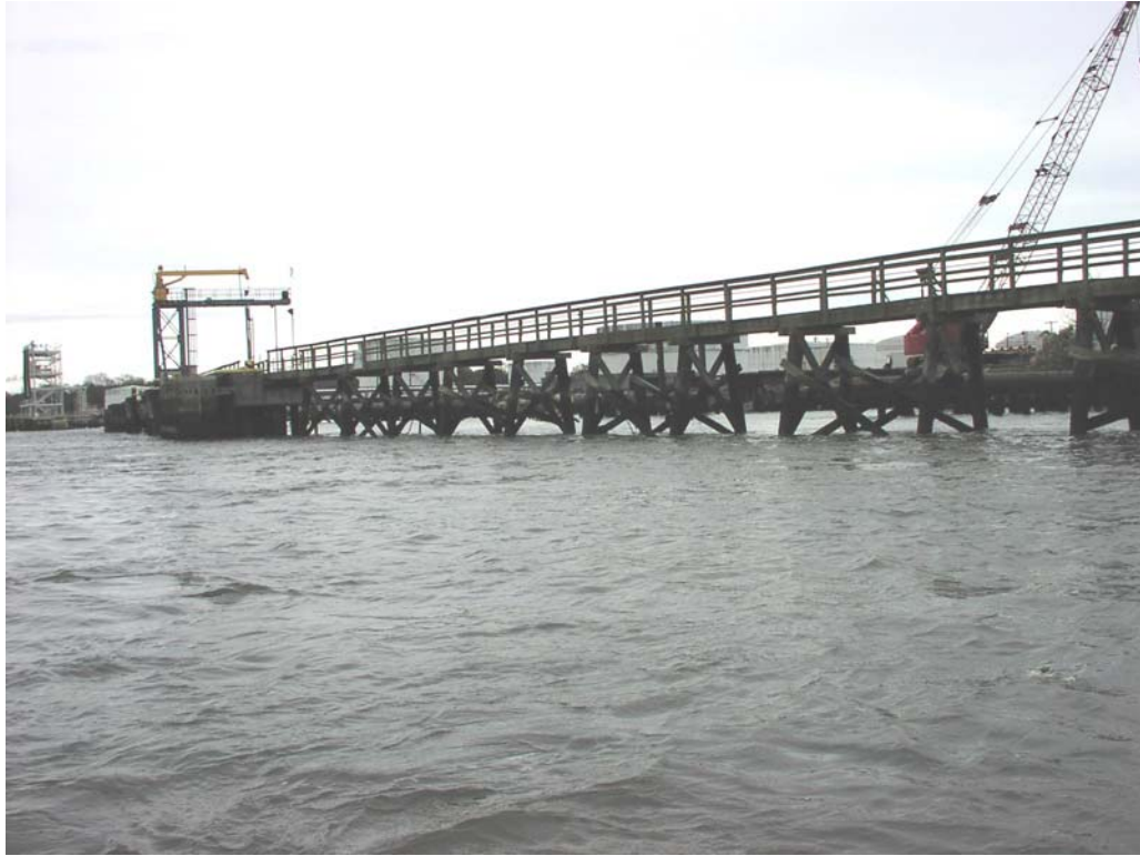
ST Services #2, Station 62+200 to 61+800, Wood/Steel Piling, Good Condition
