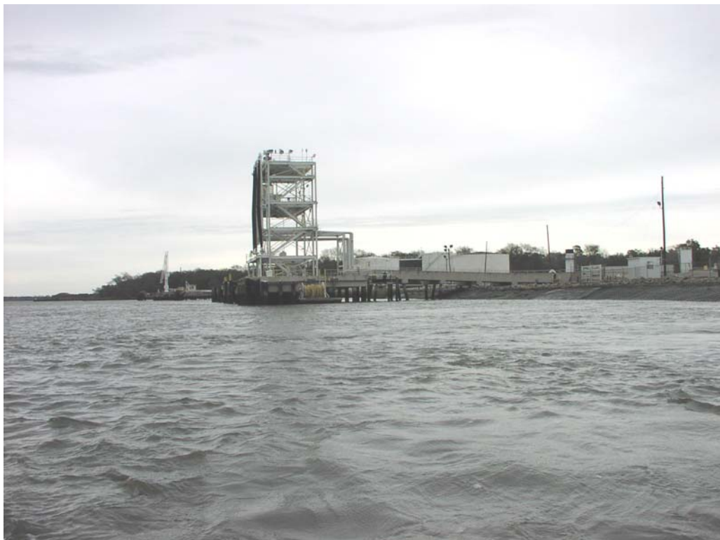
Unocal, Station 61+500, Concrete Piling, Good Condition
