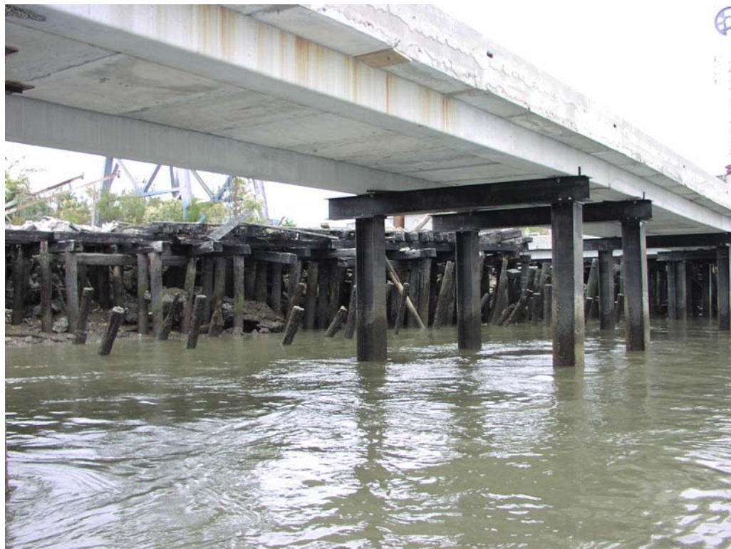
Georgia Pacific Gypsum, Steel Piles, Station 63+000, Good Condition
