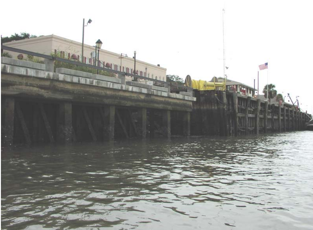
River Walk/Savannah Electric, Concrete Piles, Station 72+800, Good Condition
