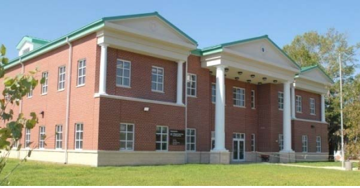
Savannah District is the CoS for Brigade Headquarters facilities, such as this 1 st BCT HQ at Fort Stewart.
