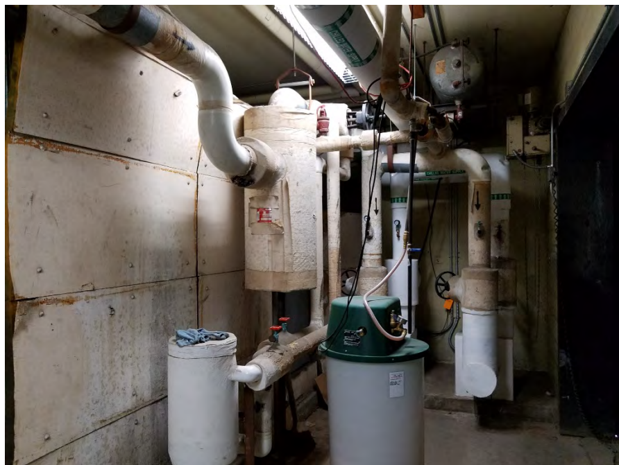
91. Distribution pipes with TSI
