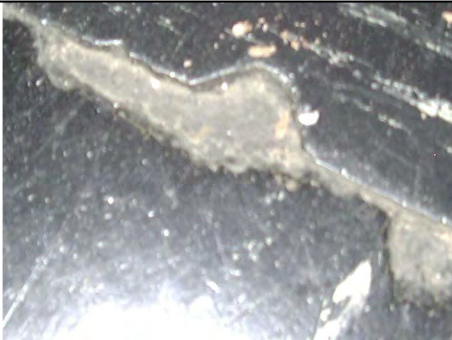
Photo 21: 9" x 9" black vinyl floor tile/ mastic– AFRC Building (Tile is Non-ACM, Mastic is positive for Asbestos)
