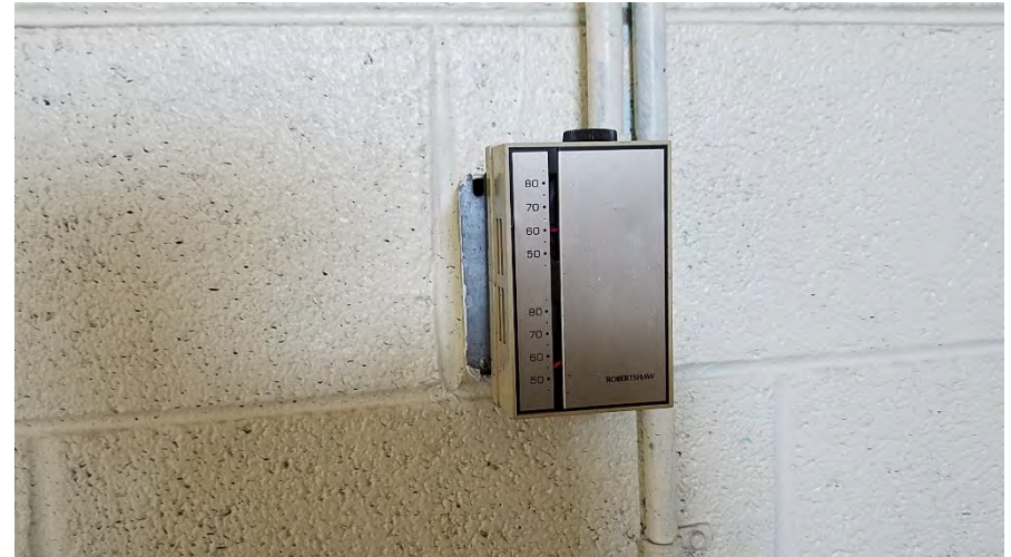
52. Old thermostat containing mercury switch located inside the OMS
