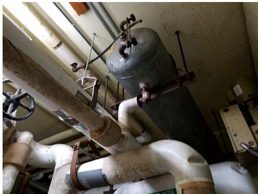
92. Distribution piping and holding tank near the ceiling inside the HVAC room
