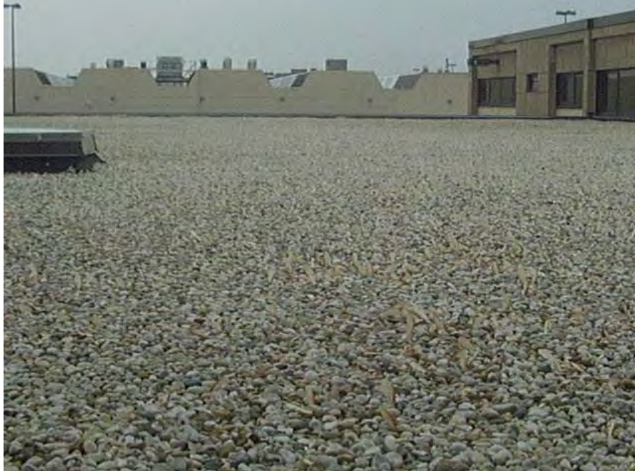
Photo 16: Roofing material- AFRC Building (Non-ACM)
