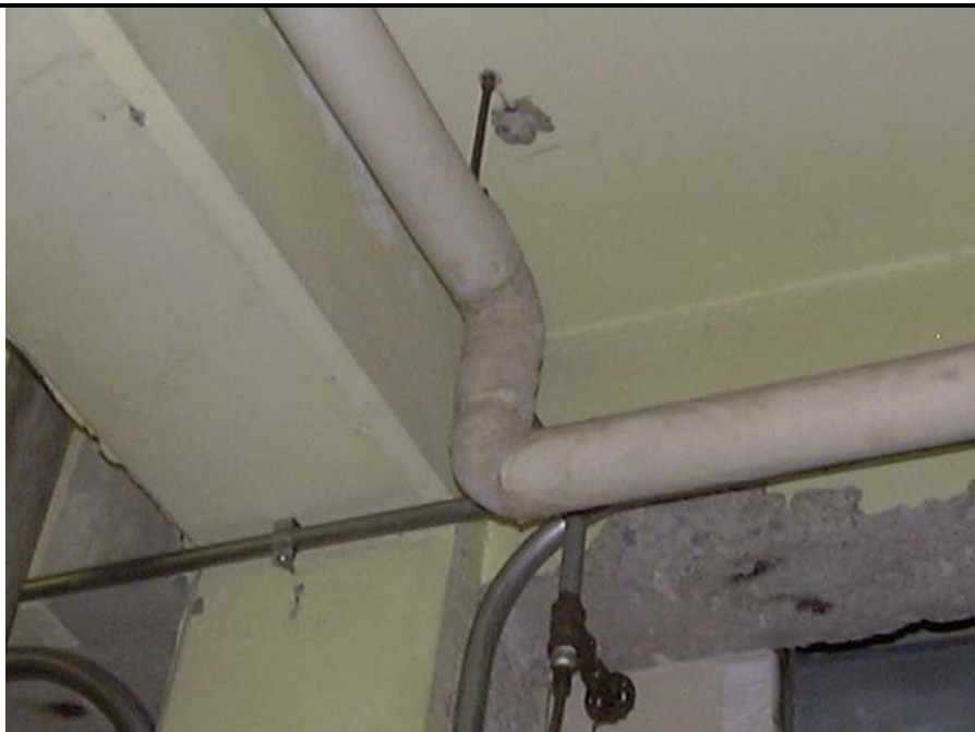
Photo 14: Paper on fiberglass insulation - OMS Building (Non-ACM)
