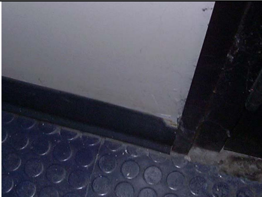
Photo 3: black vinyl baseboard/ mastic– AFRC Building (Non-ACM)
