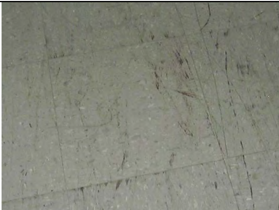
Photo 5: 12" x 12" gray vinyl floor tile/ mastic - AFRC Building Rooms 121 and 122 (Top Layer Tile and Mastic, Bottom Layer Tile is Non-ACM, Bottom Layer Mastic is positive for Asbestos)
