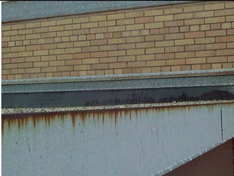
Photo 17: Roof caulk- AFRC Building (Non-ACM)
