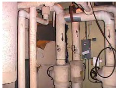
Thermal System Insulation (Non ACM)
