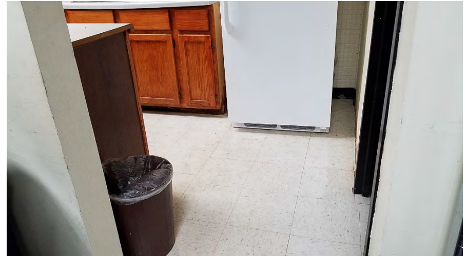
34. 9-inch x 9-inch tile flooring in the kitchen. Mastic contains non-friable ACM (2006 ECP Report)
