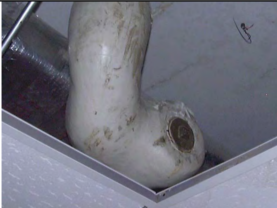
Photo 19: 12" drain pipe insulation- AFRC Building (Insulation Positive for ACM)
