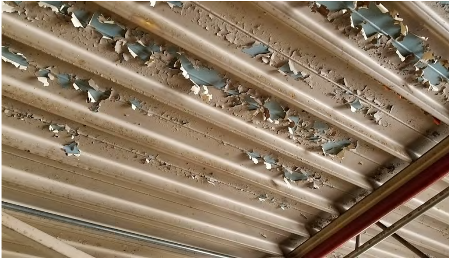
55. Peeling paint from the metal ceiling of the OMS. Based on the age of the building, the paint may contain lead
