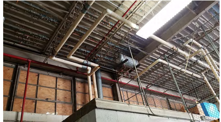
56. Another view of the ceiling with peeling paint. HVAC piping and fluorescent lighting
