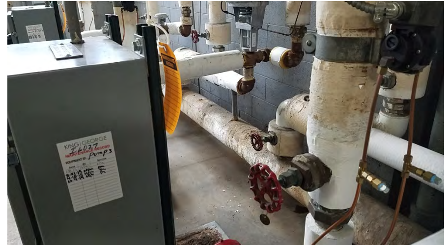
86. TSI on water distribution lines
