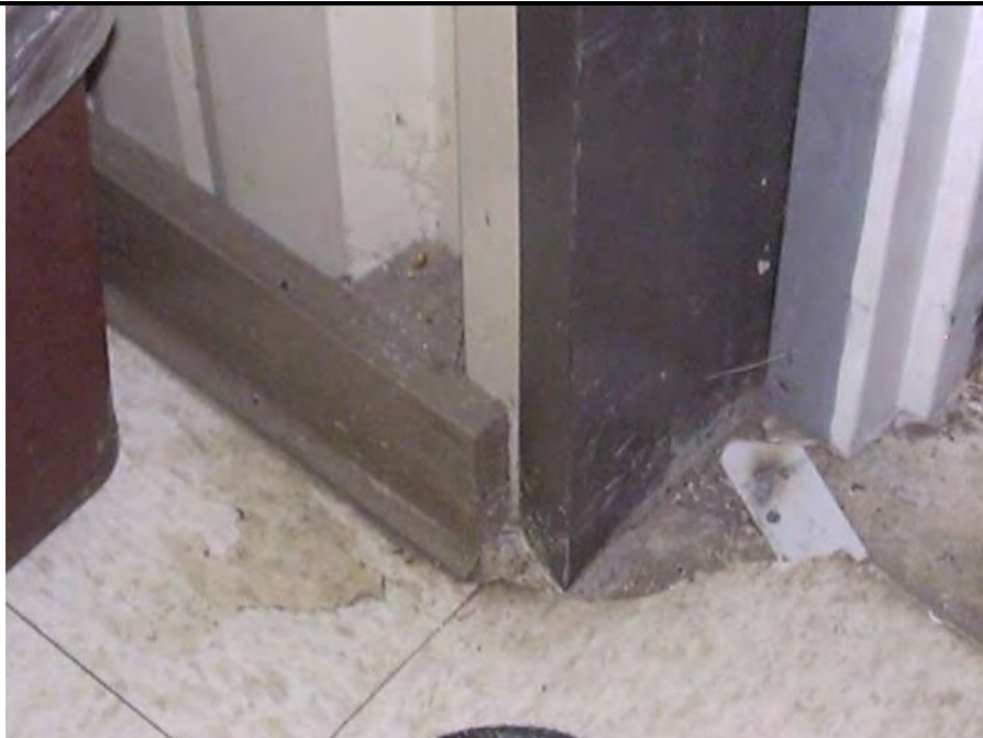
Photo 9: Blue vinyl baseboard/ mastic – AFRC Building (Non-ACM)
