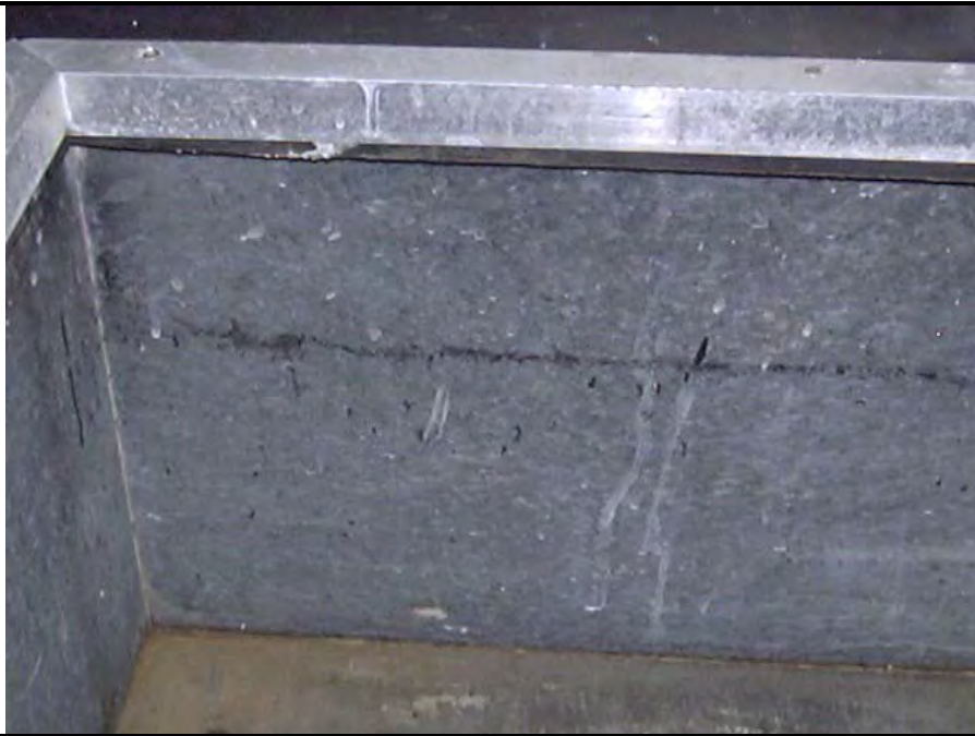
Photo 23: Transite sink- AFRC Building Room 261 (Presumed ACM)
