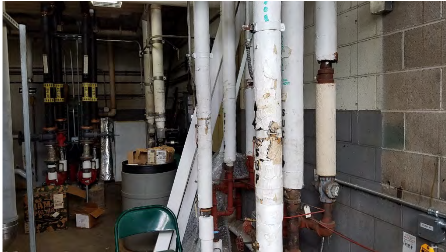
85. Damaged TSI in the boiler room
