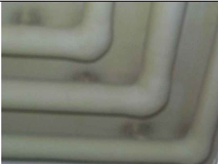
Photo 18: 2" pipe elbow insulation- AFRC Building (Insulation Positive for ACM)
