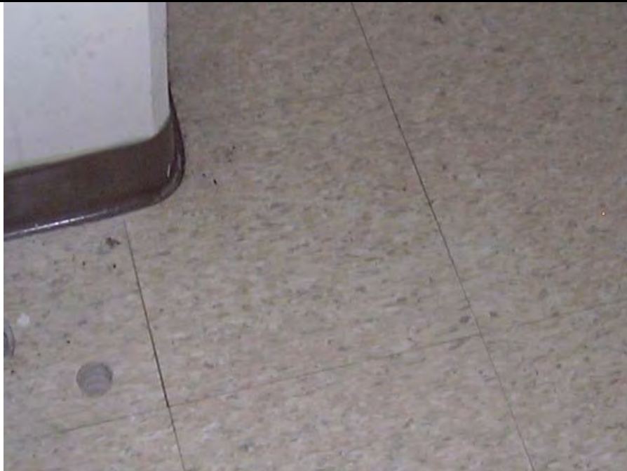
Photo 5: 12" x 12" gray vinyl floor tile/ mastic - AFRC Building Rooms 121 and 122 (Top Layer Tile and Mastic, Bottom Layer Tile is Non-ACM, Bottom Layer Mastic is positive for Asbestos)
