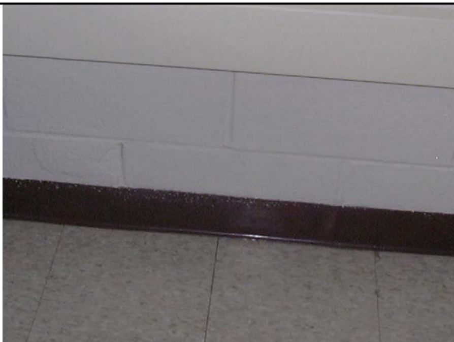
Photo 10: Brown vinyl baseboard/ mastic– AFRC Building (Non-ACM)
