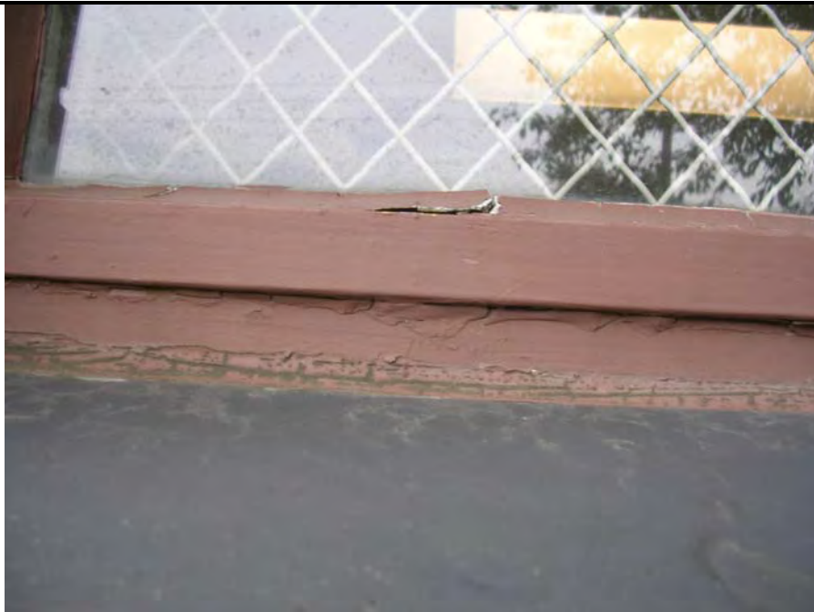
Photo 15: Window caulk-OMB Building ( Caulk is positive for Asbestos )
