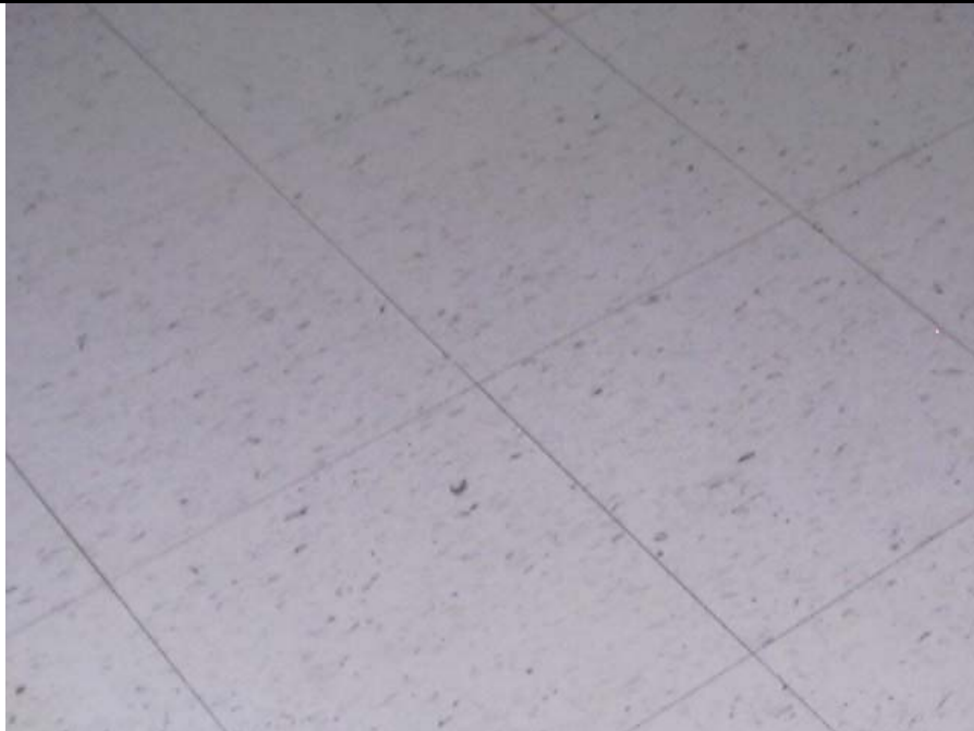
Photo 11: 12" x 12" off-white vinyl floor tile/ mastic– AFRC Building (Tile is Non-ACM, Mastic is positive for Asbestos)
