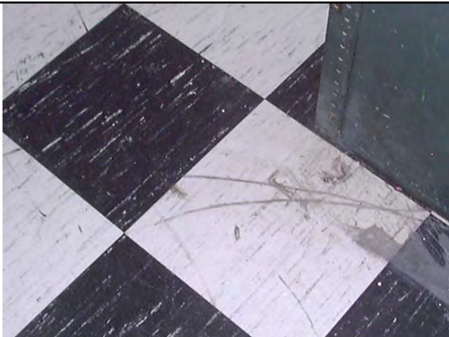
Photo 2: 12" x 12" black vinyl floor tile/ mastic– AFRC Building (Tile is Non-ACM, Mastic is positive for Asbestos)
