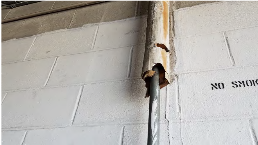
49. Damaged pipe insulation inside the OMS
