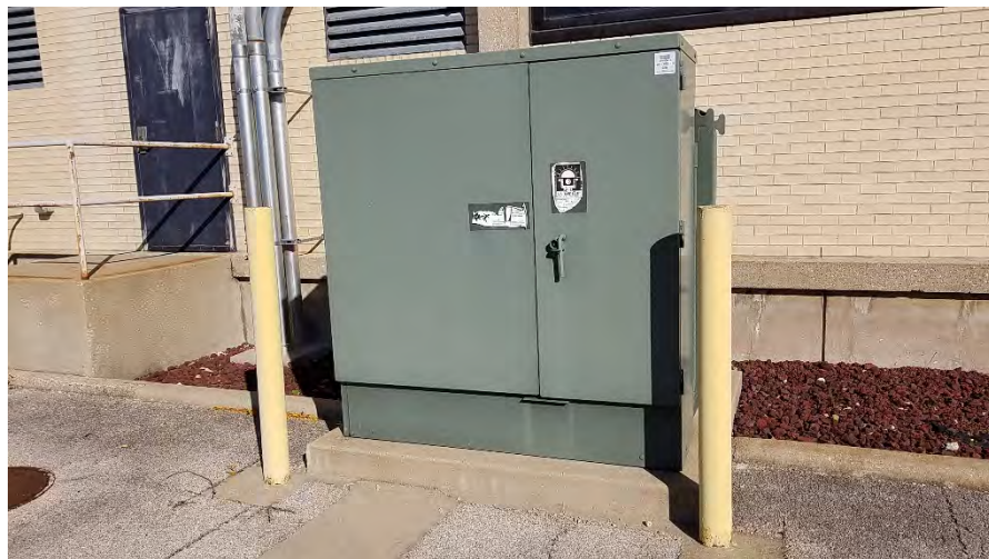
7. Pad mounted transformer – south side of the AFRC Building
