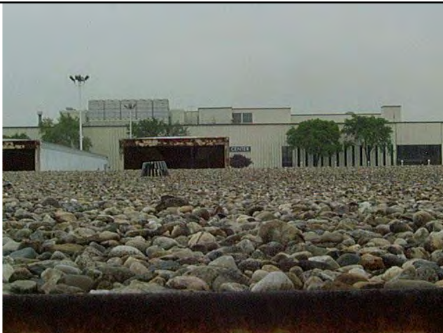
Photo 22: Roofing material - OMS Building (Non-ACM)
