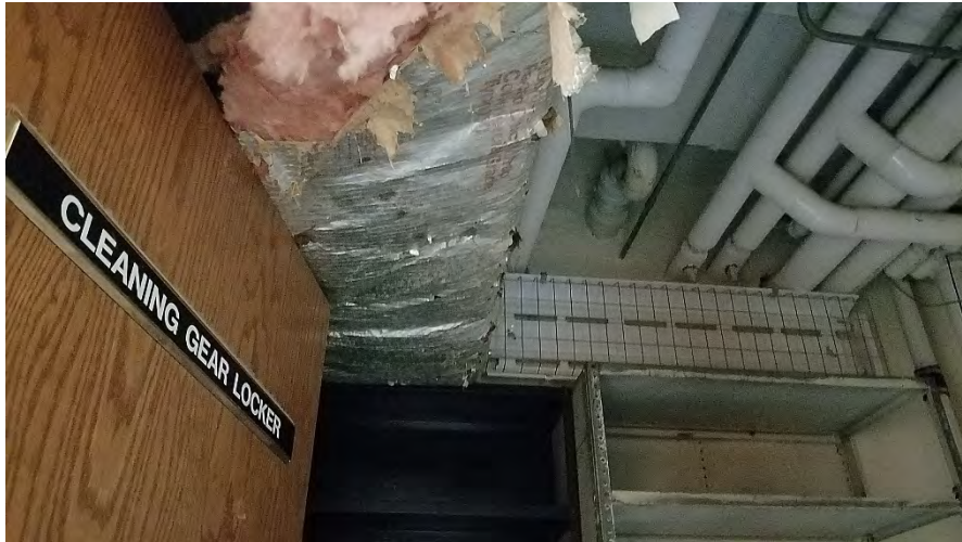
25. Exposed insulation in a HVAC duct and utility pipes in the ceiling of a cleaning supplies storage room
