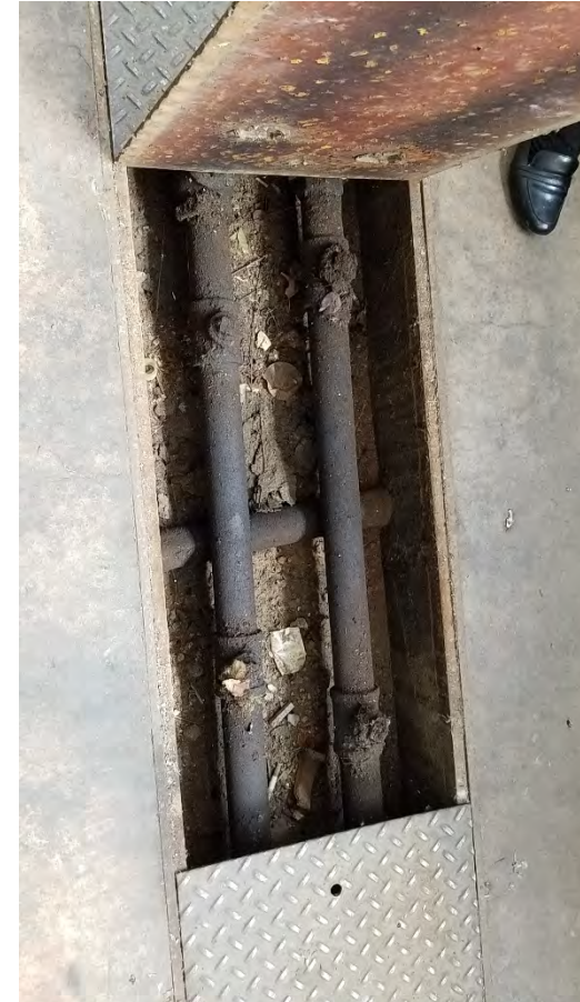
88. Piping in the utility trench inside the boiler room
