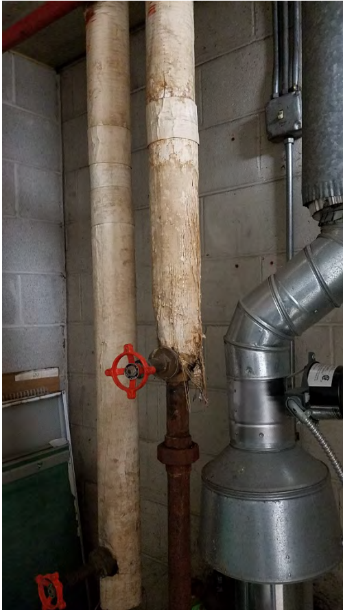
81. Damaged Thermal System Insulation (TSI) in the boiler room in the Admin Building
