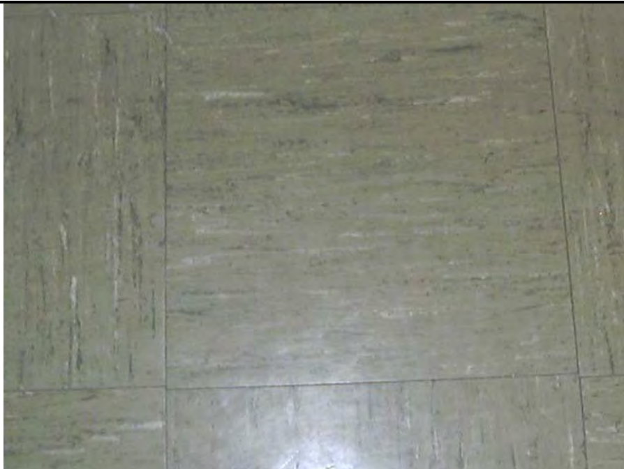
Photo 1: 12" x 12" green vinyl floor tile/ mastic – AFRC Building (Tile is Non-ACM, Mastic is positive for Asbestos)
