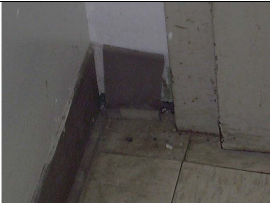
Photo 8: Gray vinyl baseboard/ mastic– AFRC Building (Non-ACM)
