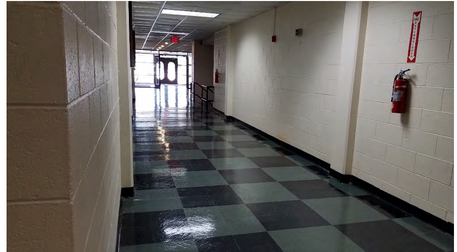
24. Another corridor in the AFRC Building. Green and black colored tiled flooring contains non-friable asbestos containing material (ACM)
