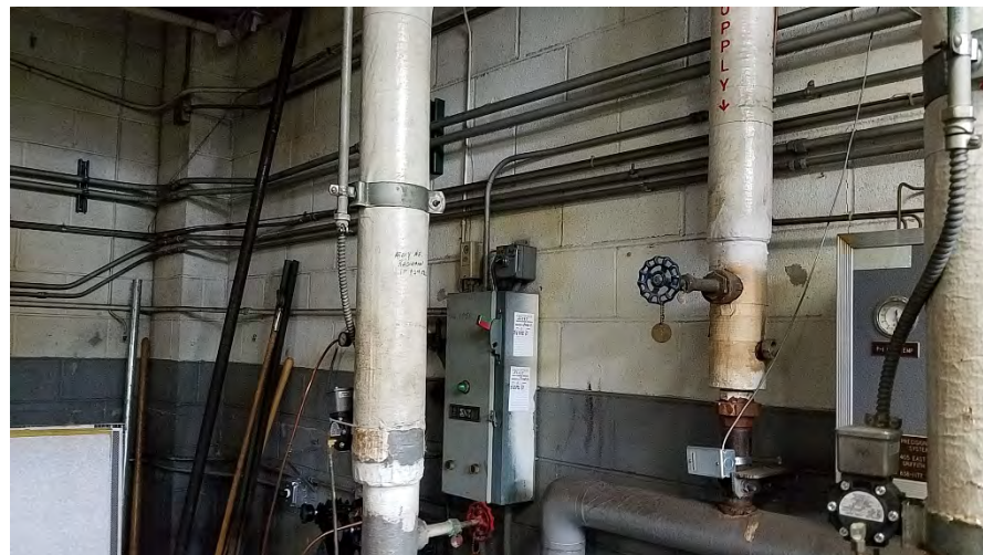
84. Piping wrapped with TSI
