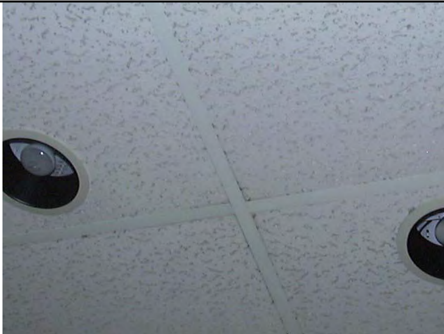
Photo 7: 2' x 2' white lay-in ceiling tile– AFRC Building (Non-ACM)
