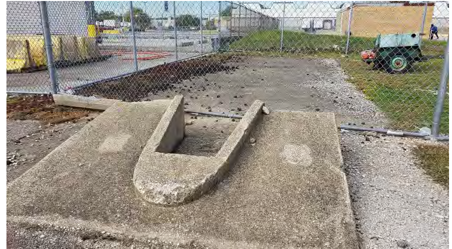
46. Ramp for accessing military vehicle's underbody for performing maintenance activities
