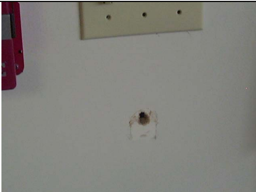
Photo 12: Plaster – AFRC Building (Non-ACM)
