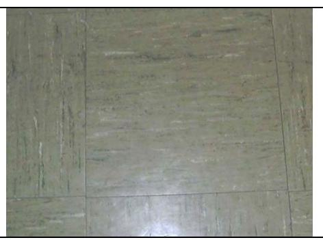
Photo 1: 12" x 12" green vinyl floor tile/ mastic (Tile is Non-ACM, Mastic is positive for Asbestos)
