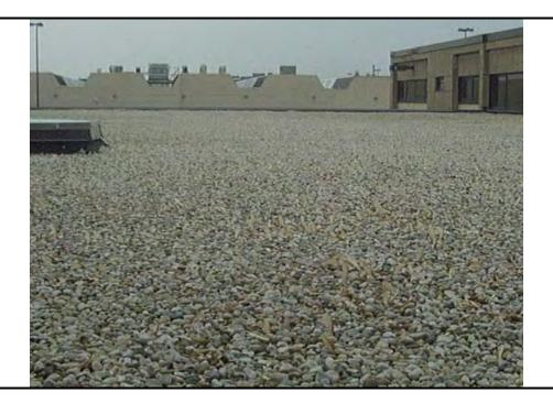
**Photo 16:** Roofing material- AFRC Building (Non-ACM)
