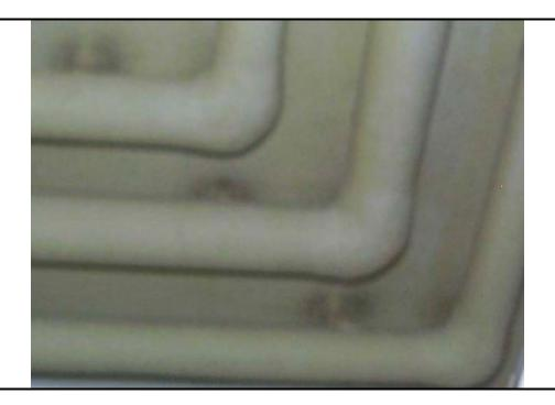
Photo 18: 2" pipe elbow insulation (Insulation Positive for ACM)
