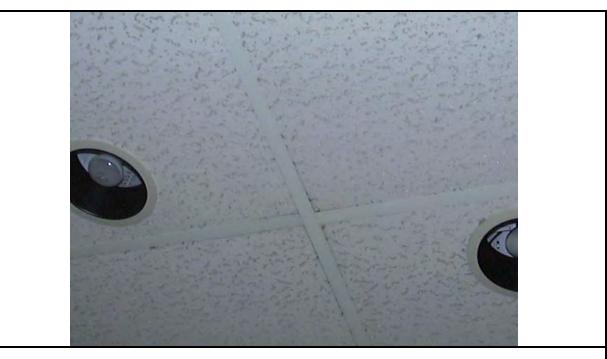
Photo 7: 2' x 2' white lay-in ceiling tile— AFRC Building (Non-ACM)
