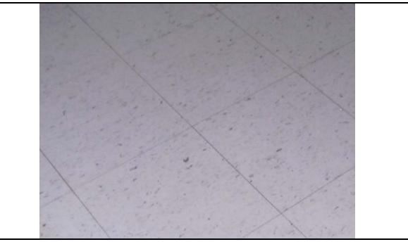
Photo 11: 12" x 12" off-white vinyl floor tile/ mastic— AFRC Building (Tile is Non-ACM, Mastic is positive for Asbestos)
