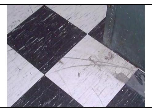
Photo 2: 12" x 12" black vinyl floor tile/ mastic (Tile is Non-ACM, Mastic is positive for Asbestos)
