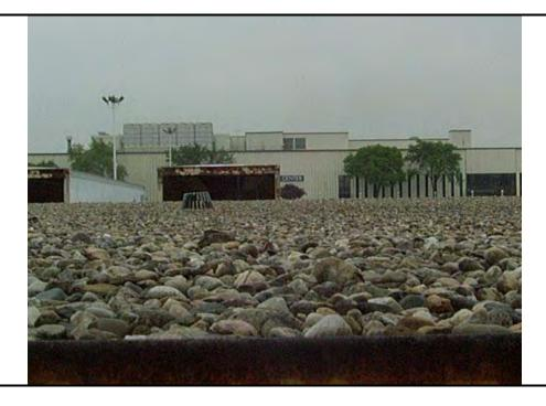
Photo 22: Roofing material - OMS Building (Non-ACM)
