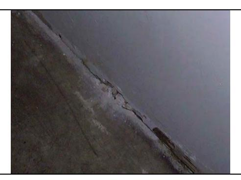
Photo 13: Drywall/ joint compound (Non-ACM)
