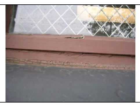
Photo 15: Window caulk (Caulk is positive for Asbestos)
