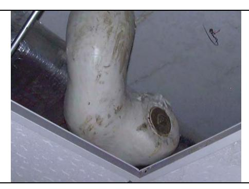
Photo 19: 12" drain pipe insulation (Insulation Positive for ACM)
