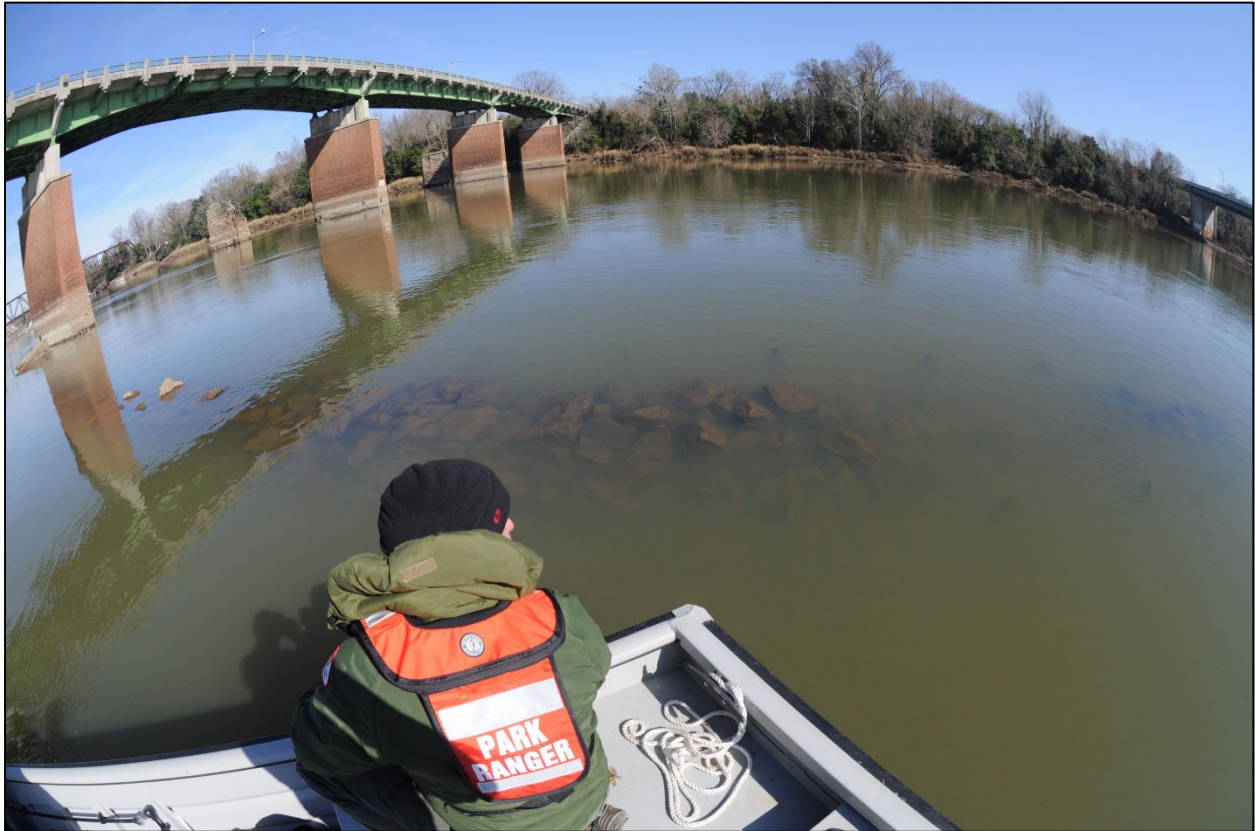
Figure 2. Photograph of submerged training wall
