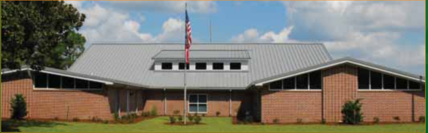
The GPA has applied for LEED Commercial Interiors (CI) Silver status for the Annex 2 building. Reflective materials were used for roof construction to increase the building's overall energy efficiency by reducing the interior heat load.
