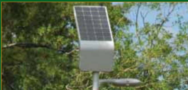
The employee parking lot features solar-powered lighting with no connection to the power grid.
