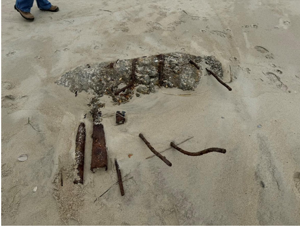
Photo 9 - One of two reinforced concrete structures located in footprint of former Building 19. Believed to be access point for submarine listening equipment to exit building toward beach/water
