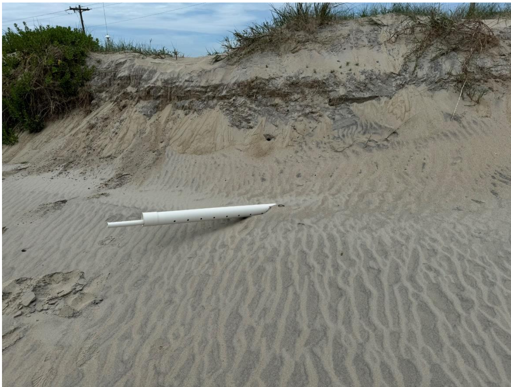
Photo 10 - Assumed sanitary leach field drain pipe located north of former Building 19.
