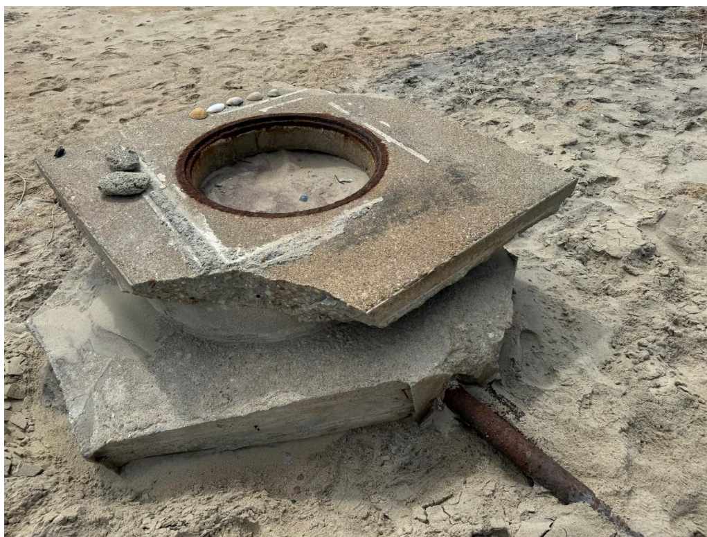
Photo 6 - Manhole structure located near southern part of former Building 19. Note two metal pipes going west from manhole.
