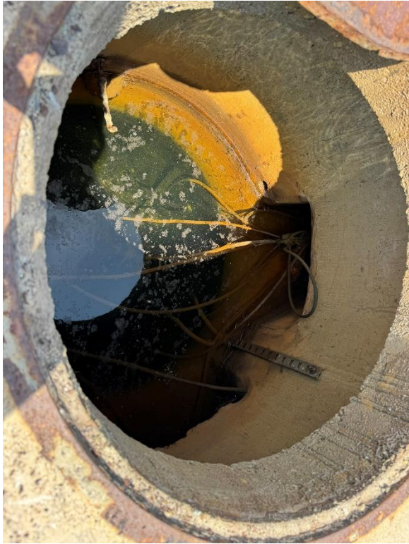
Photo 19 - One of two manholes located west of dunes, eastern/southern part of FUDS. Both contained water, no odor/sheen. Cable conduits going north-south and east-west. Assumed communication cables observed, cut-off metal pipes observed.
