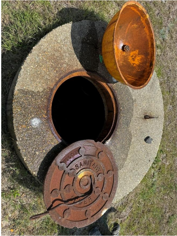
Photo 20 - One of several sanitary sewer manholes noted. Two manholes opened. No odors or sheen. One manhole had small amount of assumed groundwater baseflow
