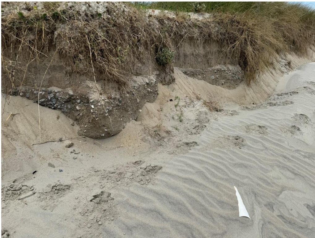
Photo 18 - Additional exposed septic leach field pipe and evidence of backfill (gravel in dune face)
