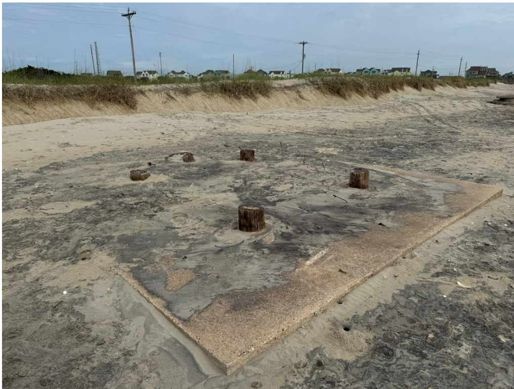
Photo 8 - Concrete pad with timber piers located south of former Building 19 and manhole structure.
