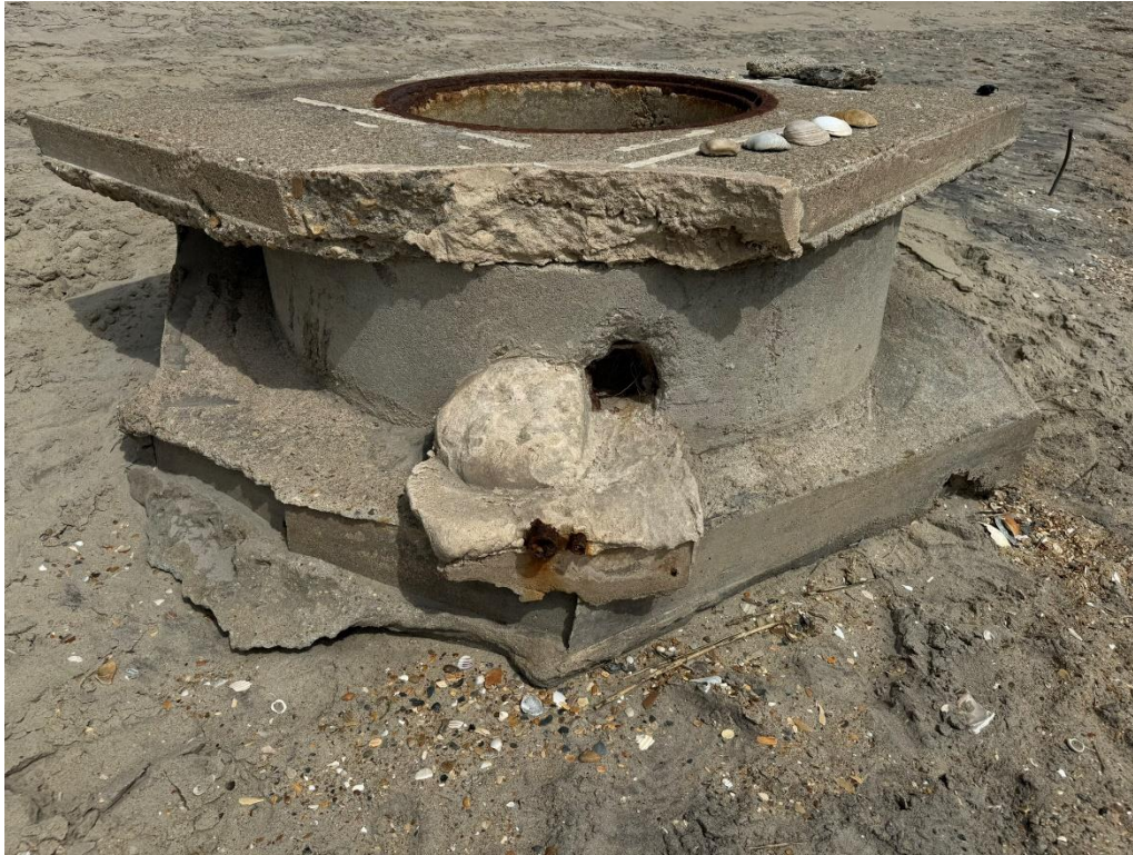
Photo 7 - Additional view of manhole structure. Two smaller pipes/conduits protruding to southeast. Smaller conduit appears to have metal cable inside.
