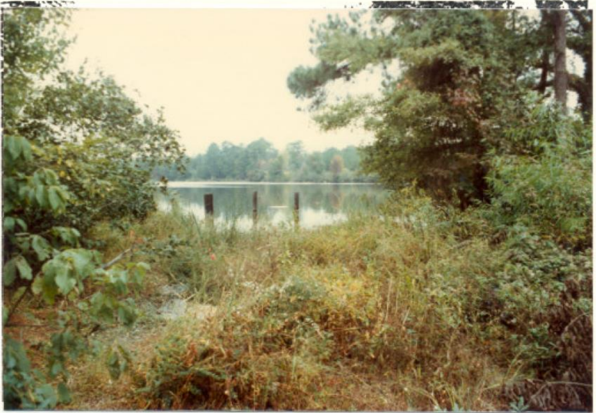
Photo 7 : Spillway entrance viewed from spillway channel
