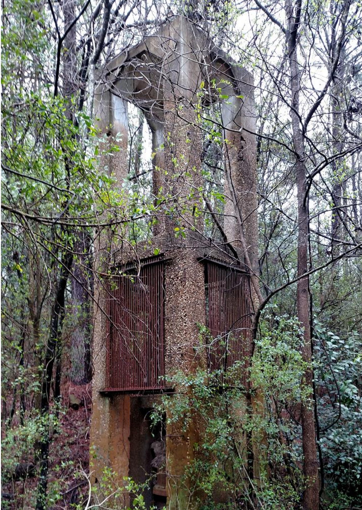
Photo 9 : Old Outlet Structure
