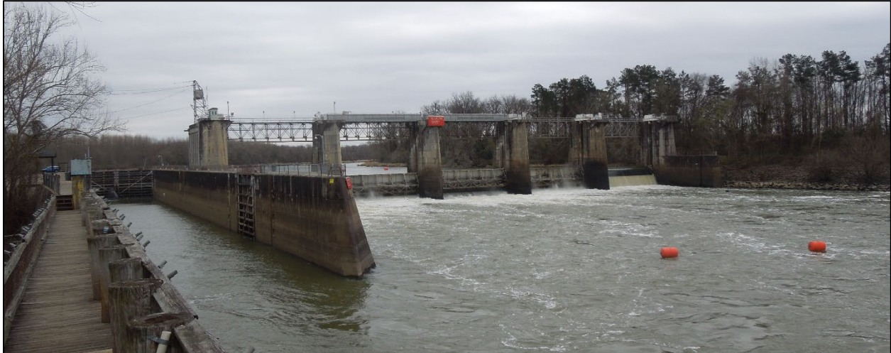
Figure 1 - New Savannah Bluff Lock and Dam - viewpoint looking upstream from the Georgia side.
