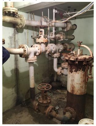
Photo 7: Piping of Original Hydraulic System located in Basement Area
