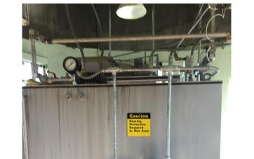
Photo 3: New Hydraulic Oil Tank located inside Lock and Dam Control Room
