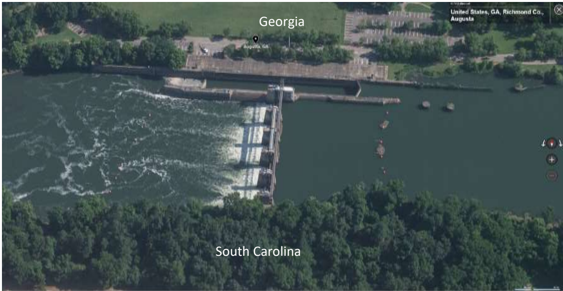
Figure 2: Bird’s Eye View of current conditions at New Savannah Bluff Lock and Dam.
