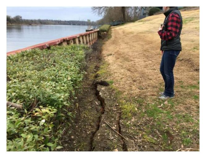
As a result of this evaluation USACE made the decision to cancel the remainder of the simulation to alleviate some of the pressure on the retaining wall. Operators at Thurmond Dam immediately began bringing the pool back up to normal operations.
