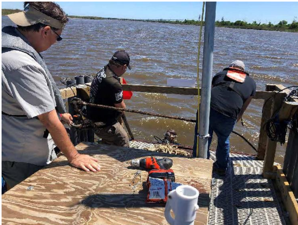
Photo 4 – Southeast Manta ray anchor being extracted from river.
