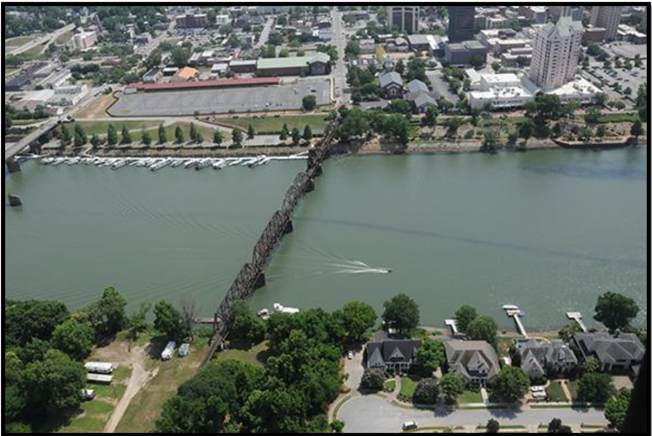
View from South Carolina of the Training Wall Centerline of the Savannah River
