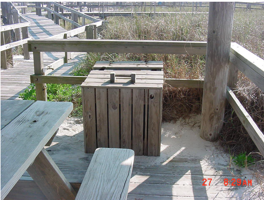
Example of trash receptacle must be secured or heavy enough so it is not easily turned over.
