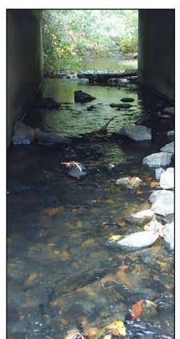
The culvert is installed at a relatively flat gradient to allow substrate to colonize the culvert's
