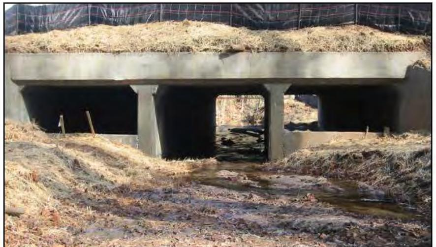
The culvert is installed at a relatively flat gradient to allow substrate to colonize the culvert's
