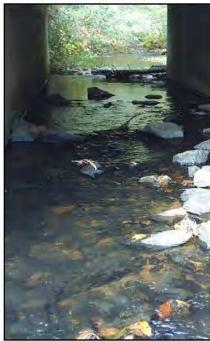
The culvert is installed at a relatively flat gradient to allow substrate to colonize the culvert's interior and maintain natural flow velocity.
