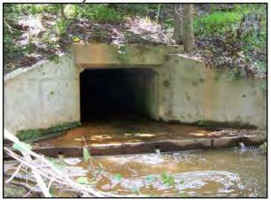
**Poorly-sized or Installed Culverts:** Undersized culverts restrict stream flow, particularly during floods. Water exits at a high velocity, causing channel and bank erosion. Overly-wide culverts spread stream flow out so depths are too shallow for many fish and other aquatic organisms to swim or move through.
