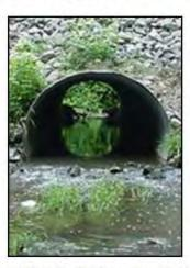
Bottomless or embedded culverts wide enough to carry baseflows without altering stream depth (i.e., width equal to or slightly greater than the average channel width).
