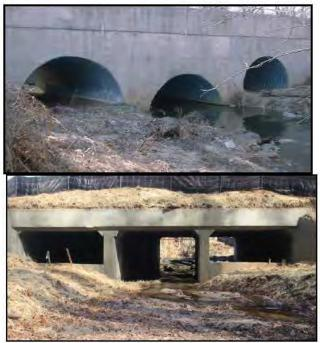
Culverts, set at bankfull elevation (top) or with baffles constructed at bankfull height carry flood waters but do not overwiden the channel at baseflows.
