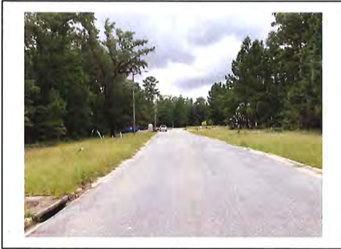
Photo 1: Typical Road Within Subdivision
