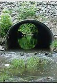
These bottomless or embedded culverts were sized so they are wide enough to carry base flows without altering stream depth (i.e., width equal to or slightly greater than the average channel width).
