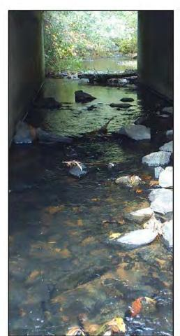
The culvert is installed at a relatively flat gradient to allow substrate to colonize the culvert's
