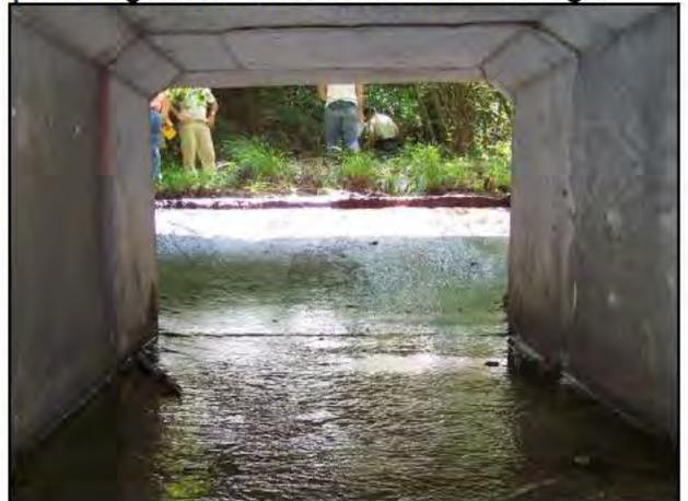
**Multiple Pipe Culverts:** Culverts with two or more widely-spaced pipes are prone to clogging, which may inhibit fish movement; increase water velocity in the remaining pipes; cause flooding into roadside ditches, resulting in problems for roadways; and cause water to scour the channel banks, causing bank erosion and increased maintenance costs.
