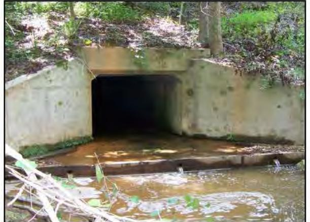
**Poorly-sized or Installed Culverts:** Undersized culverts restrict stream flow, particularly during floods. Water exits at a high velocity, causing channel and bank erosion. Overly-wide culverts spread stream flow out so depths are too shallow for many fish and other aquatic organisms to swim or move through.
