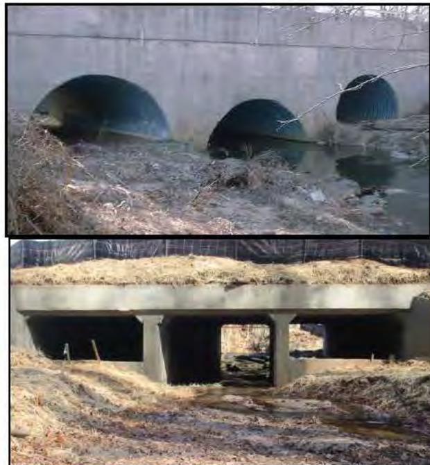
Culverts, set at bankfull elevation (top) or with baffles constructed at bankfull height carry flood waters but do not overwiden the channel at baseflows.
