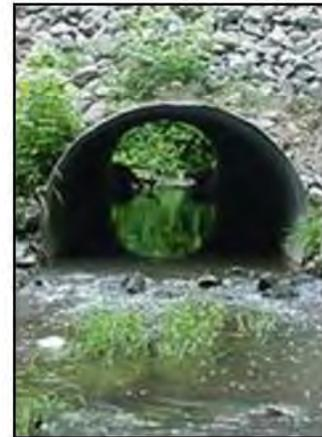
Bottomless or embedded culverts wide enough to carry baseflows without altering stream depth (i.e., width equal to or slightly greater than the average channel width).
