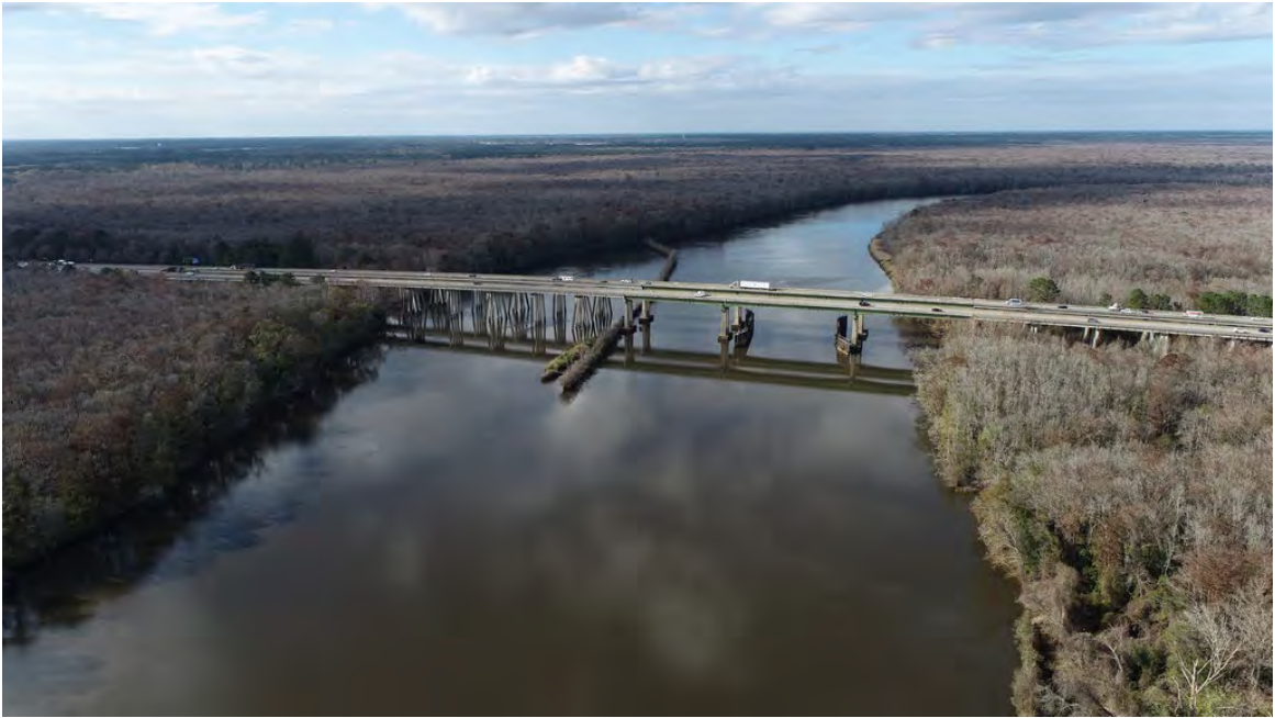
Figure 2: Upstream fender system in the project area
