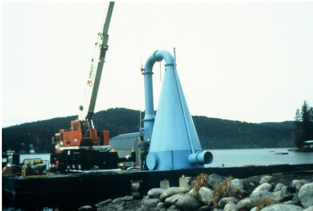
Figure 4-1 Speece Cone Being Installed in Newman Lake (from [www.eco2tech.com](http://www.eco2tech.com))
