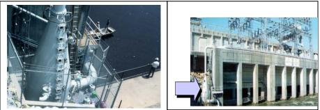
Speece Cone oxygenator and discharges about 30 foot below the tail water surface. A throttling valve is located at the discharge in the tail water to allow pressurization of the oxygenation system. This pressure corresponds to the difference in water elevation between the upstream pool and the tail water.
