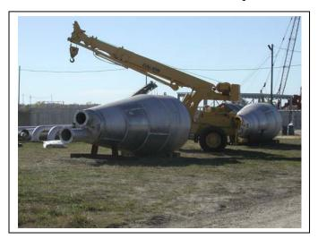
The pressure differential across the cone is rather small, being primarily in proportion to the void volume of the bubble swarm within the cone. Thus the unit energy required to pump water through the bubble swarm is relatively small, and therefore the unit energy per ton of D. O. dissolved is also relatively small.
