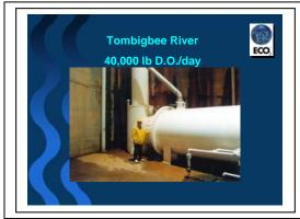
as it passes down through the U-Tube. Oxygen transfer is enhanced by the turbulence and extended contact time, but mainly by the hydrostatic pressurization as the water goes down the depth of the U-Tube and back up out the discharge. A depth of 175 feet was selected as the design depth for the U-Tube.
