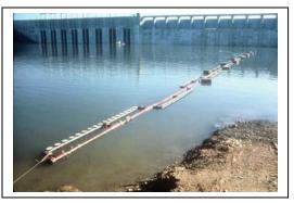
tons per day. A maximum oxygen loading rate of a hundred tons per day occurred in September and October of that year. Oxygenated water was shown to stay in the lower layer of the lake and a daily average of 6 mg/L was maintained. By the time injection was terminated in December, after the Fall turnover over 14,000 tons of oxygen had been injected.
