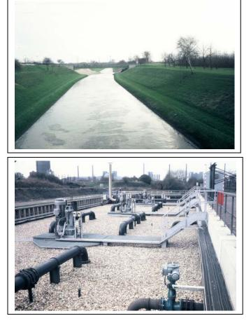
into the Rhine. However hydrogen sulfide problems in transit are an indirect effect of anaerobic processes occurring in the river. An oxygenation station is being used to remediate foul odors experienced by populations living near the river.
