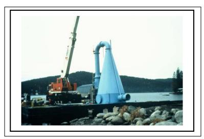
superoxygenated discharge levels. The Speece Cone can achieve O2 absorption efficiencies in excess of 90% while producing D.O. concentrations of 50 mg/L at unit
