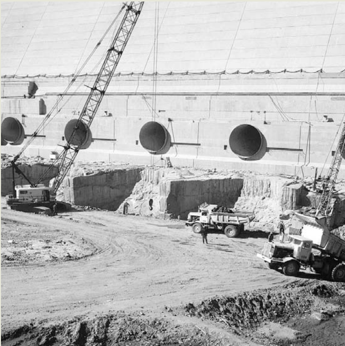
Workers build the penstocks at Hartwell Dam, the second dam and lake project the Corps constructed on the Savannah River. Construction was completed in 1962.
