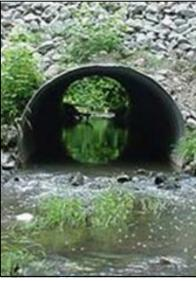
These bottomless or embedded culverts were sized so they are wide enough to carry base flows without altering stream depth (i.e., width equal to or slightly greater than the average channel width).
