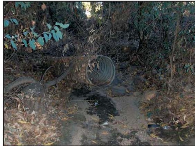
Photograph 4: Drainage A looking downstream where the 15-inch pipe is sticking out into the drainage.
