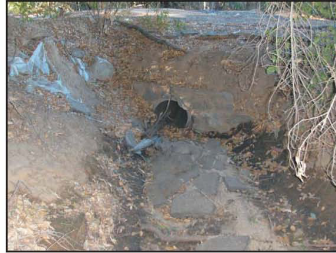
Photograph 6: Drainage A looking downstream at the 15-inch culvert along the western boundary of the Site where the drainage exits the Site.
