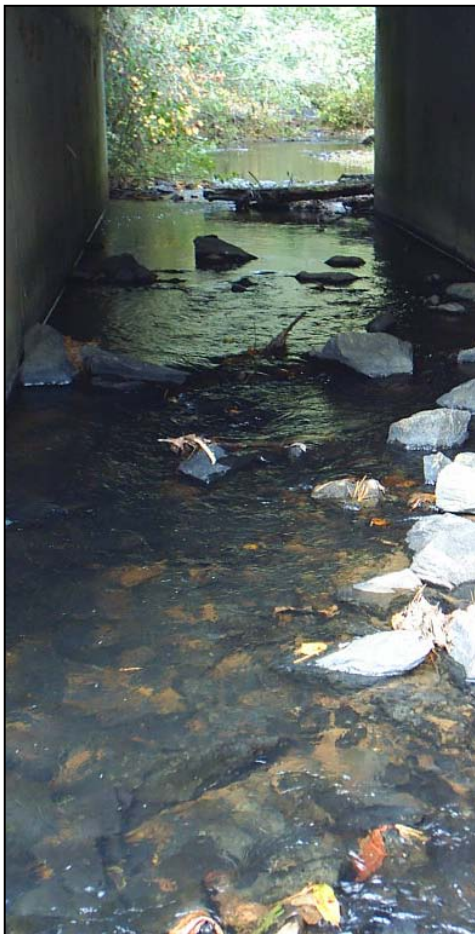
The culvert is installed at a relatively flat gradient to allow substrate to colonize the culvert's interior and maintain natural flow velocity.
