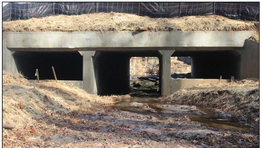
Culverts, set at bankfull elevation (top) or with baffles constructed at bankfull height carry flood waters but do not overwiden the channel at baseflow.
