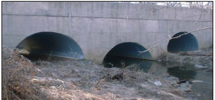
These bottomless or embedded culverts were sized so they are wide enough to carry baseflows without altering stream depth (i.e., width equal to or slightly greater than the average channel width).
