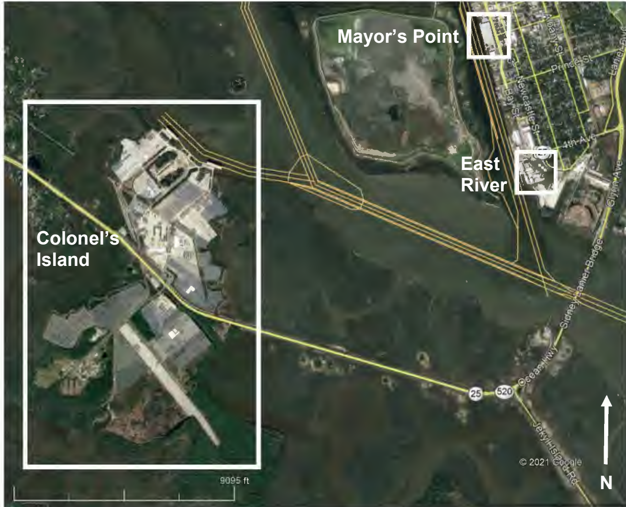
Figure 4. Brunswick Harbor Terminals
