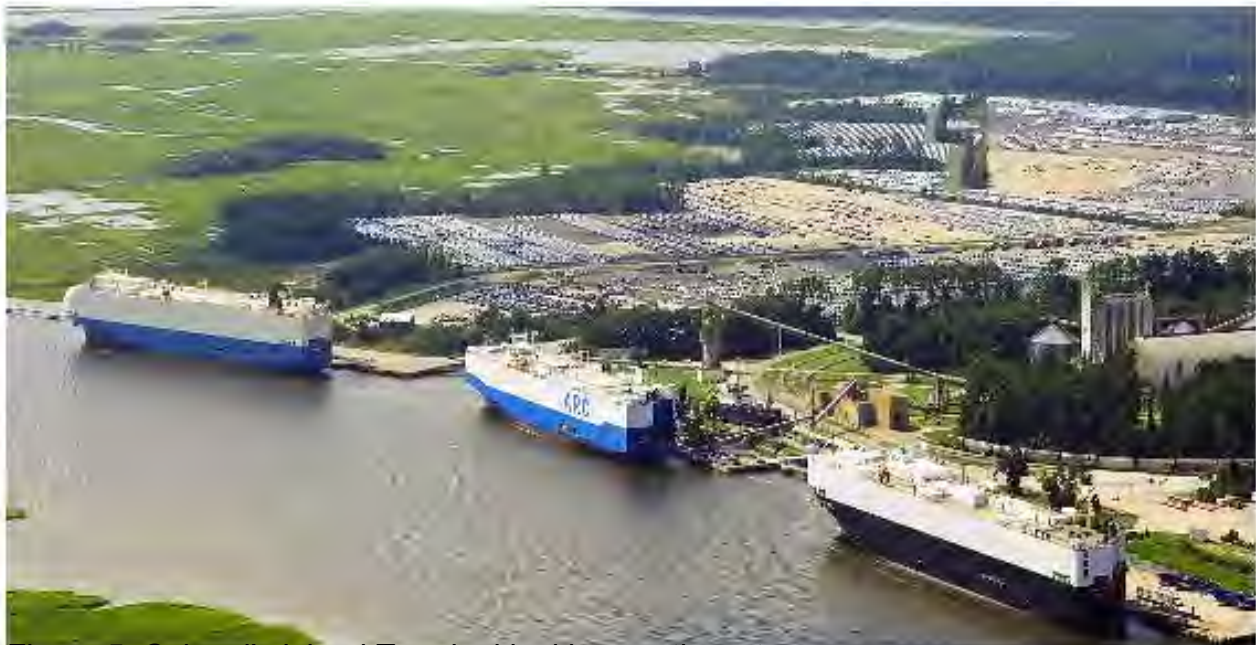
Figure 5. Colonel's Island Terminal looking southwest. Source: Georgia Ports Authority
